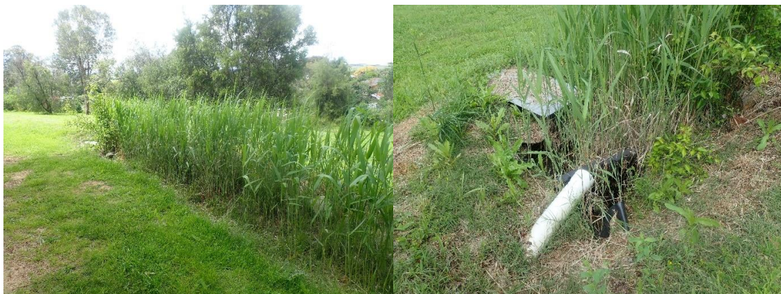
Figure 30 (left) greywater is treated in a Cumbungi wetland; (right) the pipe infrastructure needs maintenance if it is to function properly
