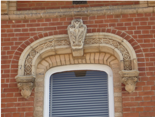
Plate 3.1.7: Decorative arch and keystone hood moulding above window over first floor window. The decorative mouldings were made at the Lithgow Pottery Works. (2007)
