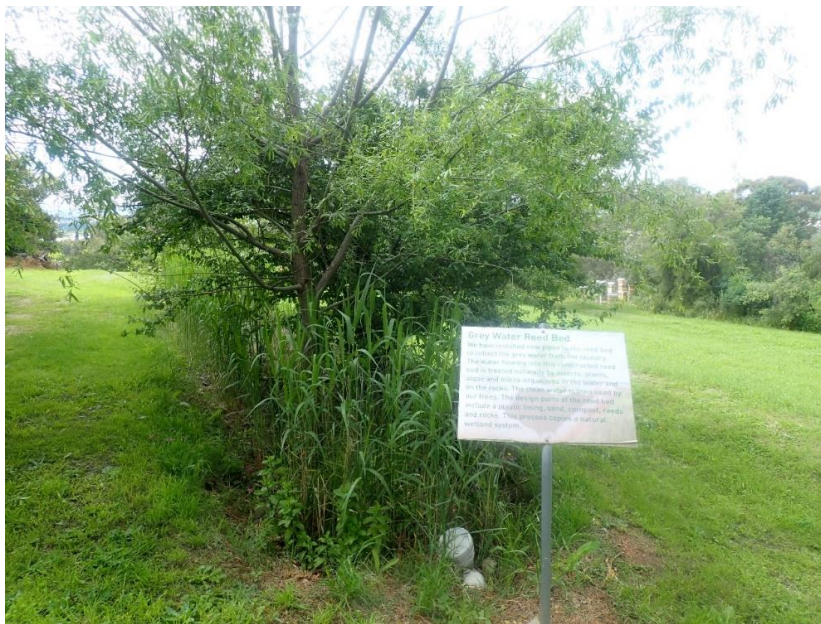
Figure 29 A greywater treatment reed bed was installed around 2010 to treat laundry water
