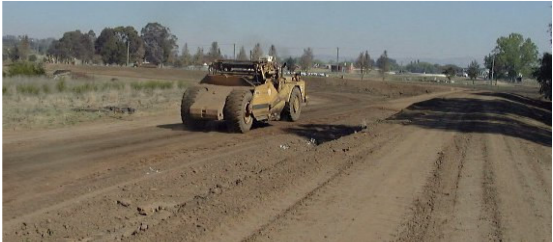
Bulk Earthworks using CAT Scrapers and Dumpsters
