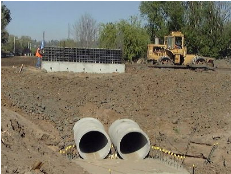
Peel Street Stormwater Outfall and Penstock Pump Pit under Construction
