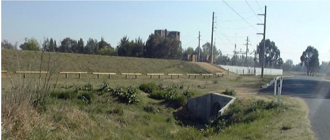
Russell Street underpass protection includes concrete levee wall to electrical substation
