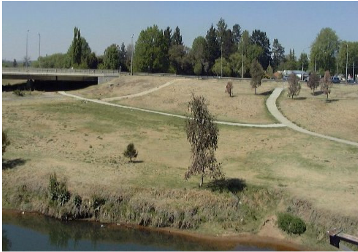
Levee constructed downstream of Evans Bridge and adjacent to Cousins Park
