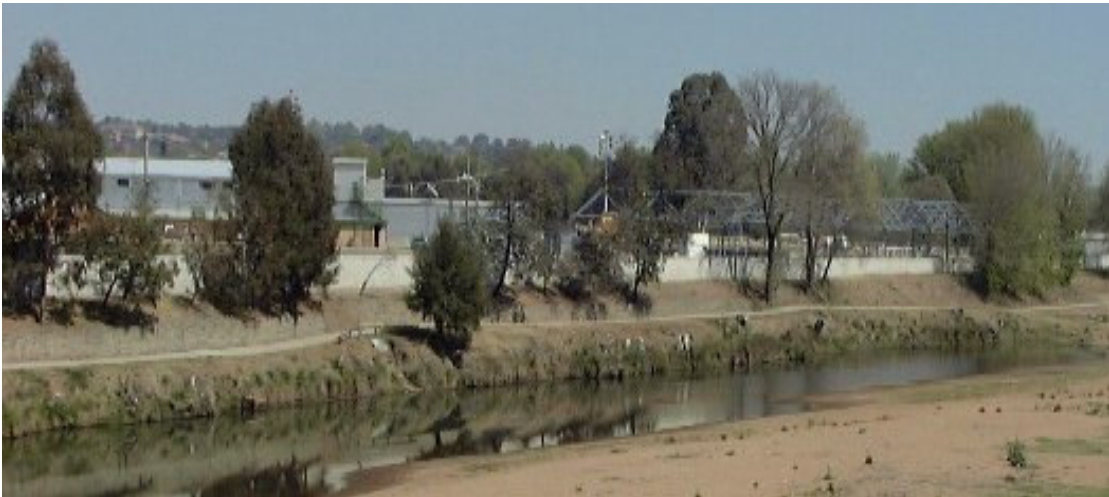
Levee wall adjacent to showground with Macquarie River in view
