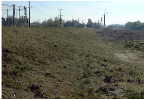
Acheron Street closed and reclaimed on levee alignment
