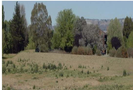
Levee constructed upstream of Evans Bridge over the Macquarie River
