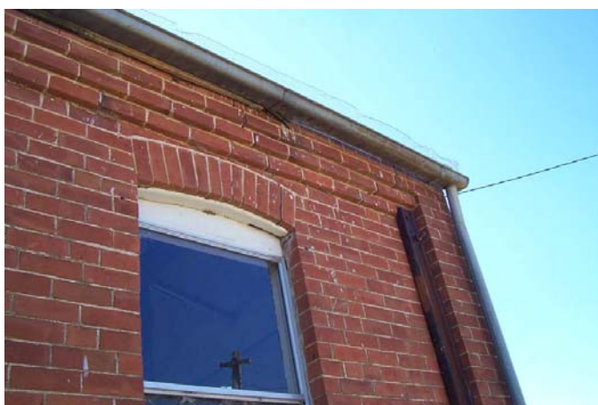
FIGURE 23 - SOUTHERN WINDOW SHOWING BRACING AND BRICK CORBELL
