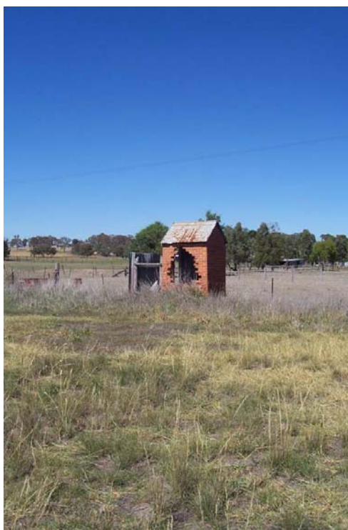
FIGURE 17 - MALE TOILET (Section of brickwork lost in Willy Willy)
