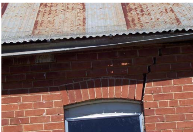
FIGURE 22 - NORTH WINDOW DETAILING CRACKING
