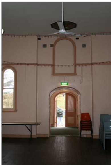
Figure 4 - Openings in Eastern Wall for Film Projection (Source: Daniel Dwyer: 2009)
