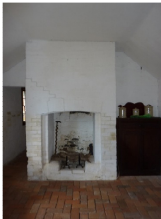
Figure 21 Most of the internal cracking has been repaired or filled. Some small cracks reappeared on chimney above. Images: BJ Hickson
