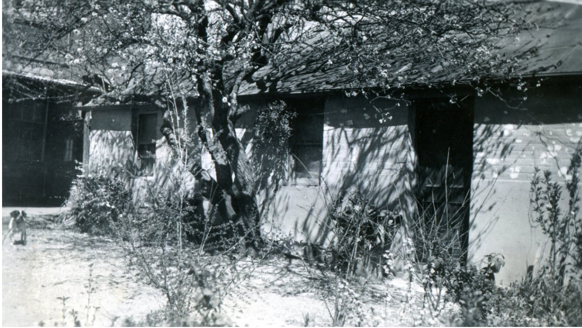
Figure 18 1958 Rutherford Image: wall detail and roof showing rendered lower section of wall and peeling or flaking paint above. Metal tiles on the roof, Courtesy BDHS
