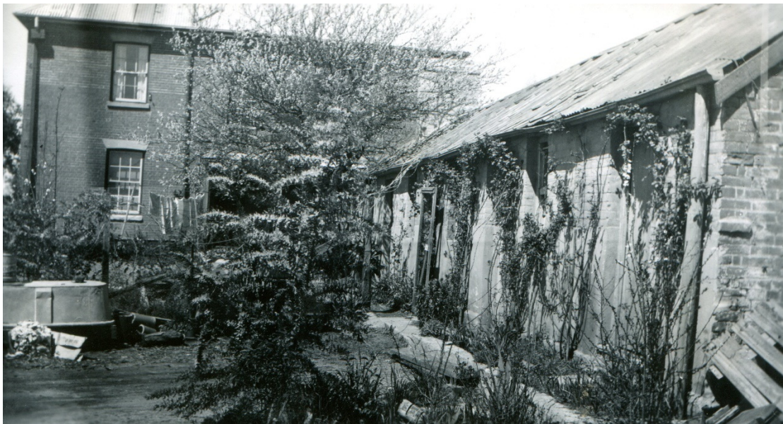
Figure 19 1958 Rutherford Image showing 1 George Street in the back ground, The poor condition of the brickwork and plants attached to the walls can be seen. Courtesy BDHS
