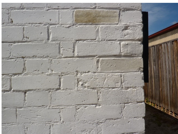
Figure 39 Detail of repointed and repainted brickwork. Image by BJ Hickson
