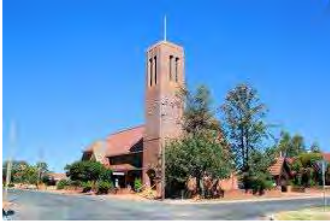
FIGURE 19 WEST WYALONG ANGLICAN CHURCH (SOURCE WWW)
