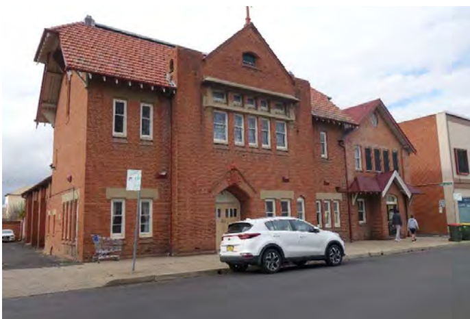
FIGURE 26 THE WALSHAW HALL BATHURST
