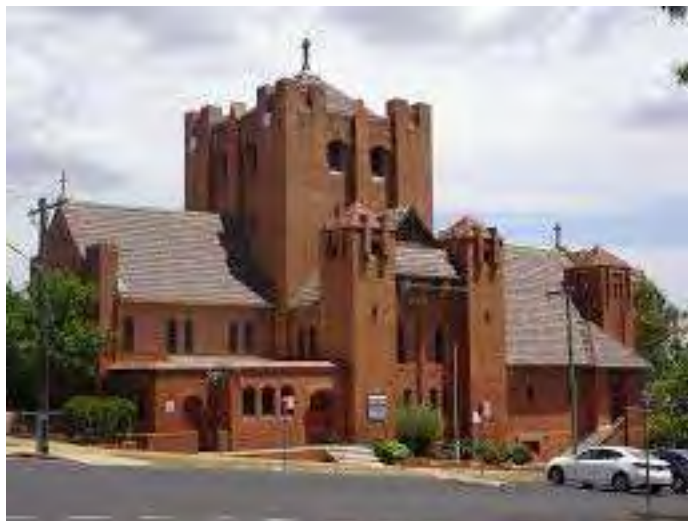
FIGURE 20 PARKES ANGLICAN CHURCH OF ST GEORGE (SOURCE SHI DATA)
