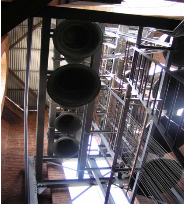
Fig. 6 The Bathurst bells were cast in the mid 1920,s and are tuned to A=435cps
