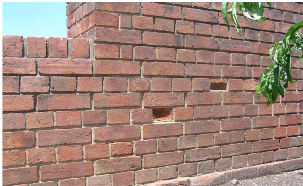
Fig. 34 details of brickwork that may be reverting to clay.
