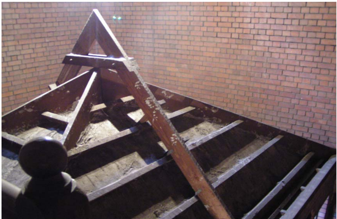
Fig. 22. The false ceiling added, possibly related to the eternal flame
