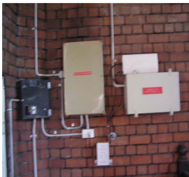
Fig. 21 Electrical system presently vulnerable to lightning strikes
