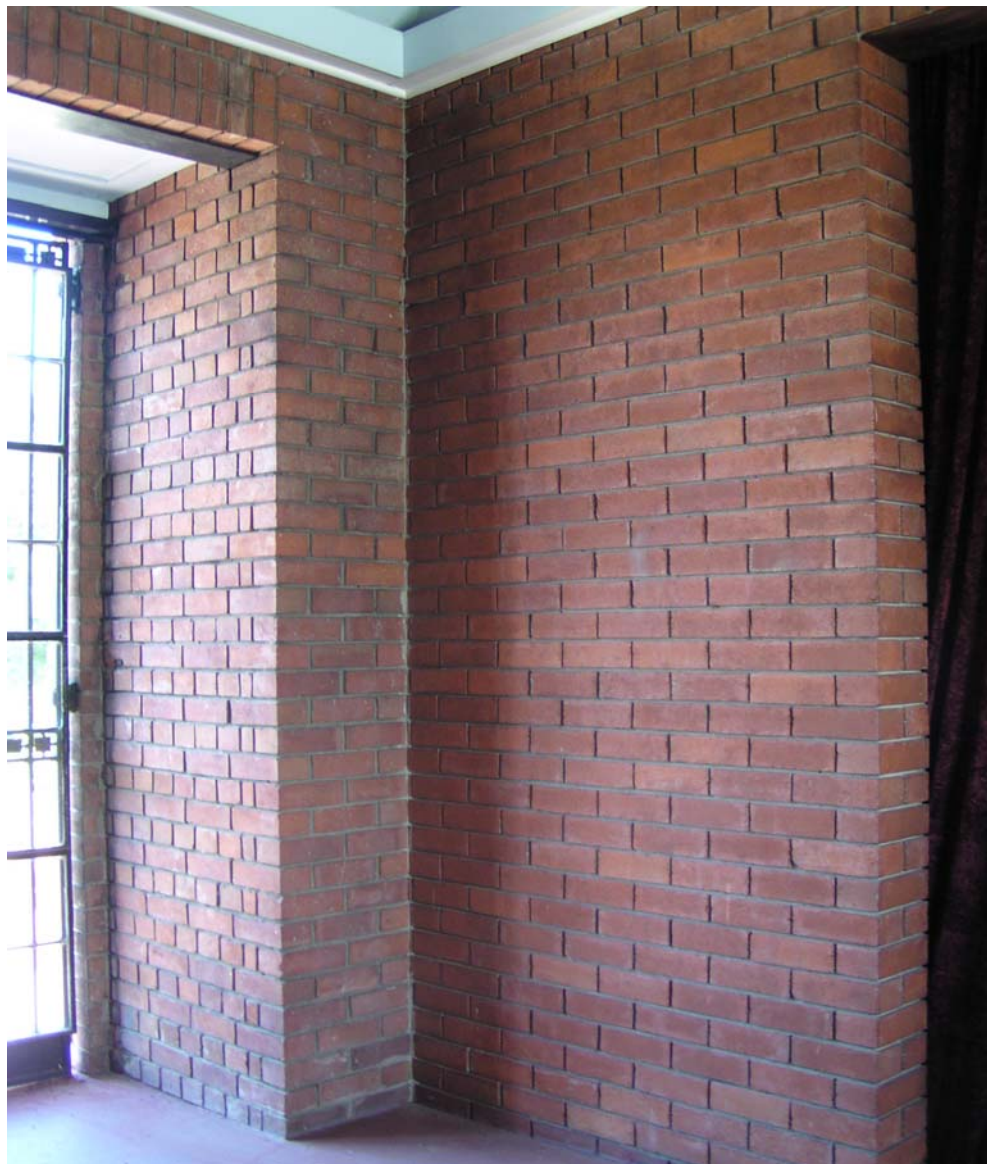
Fig.20. The Added brick blade walls. Note change from English bond to stretcher bond.
