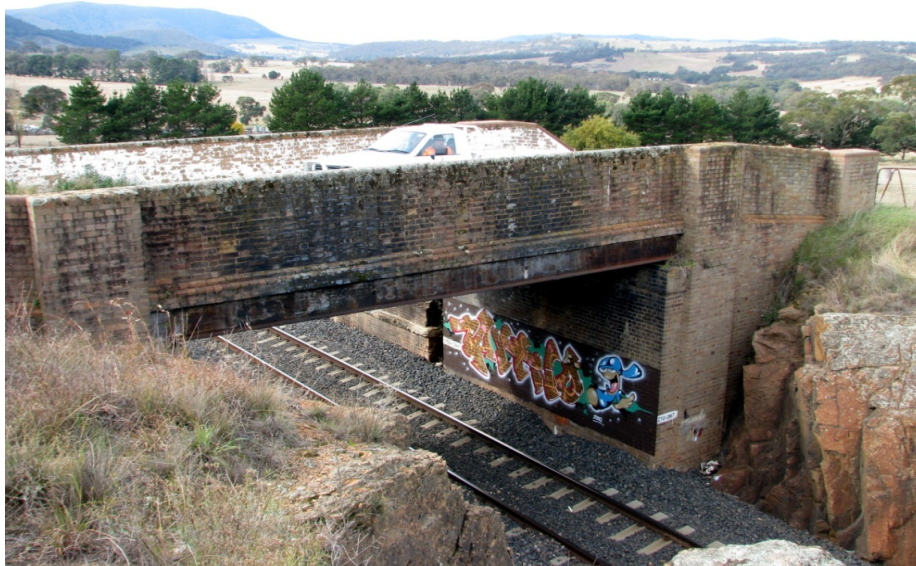
Figure 32: F82 A replacement bridge with steel frame and brick balustrade
