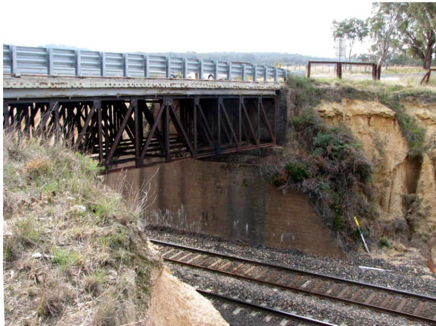
Figure 49: F77 Steel truss railway bridge over the new dual track line in 1898
