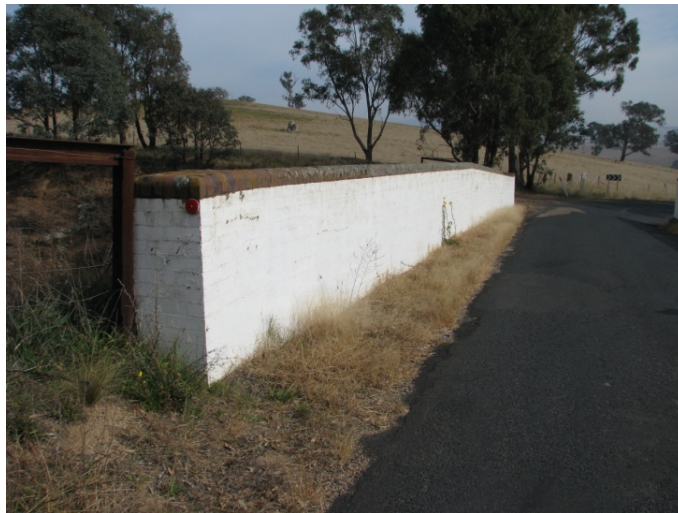
Figure 85: F73 Typical painted bridge balustrade. This bridge is a rail overpass bridge in Brewongle
