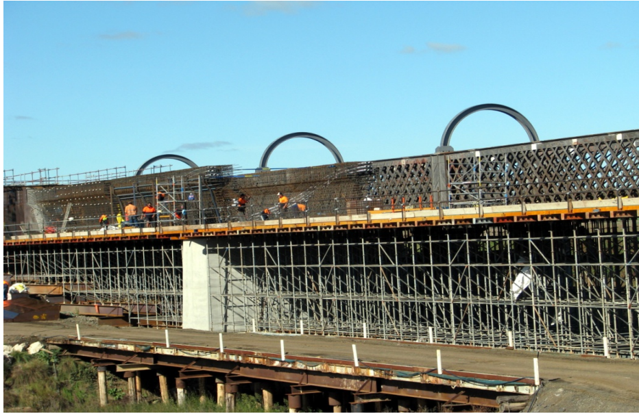
Figure 46: F63 The steel lattice girder rail bridge over the Macquarie River with a new concrete bridge under construction in the foreground (image 7 May 2010)
