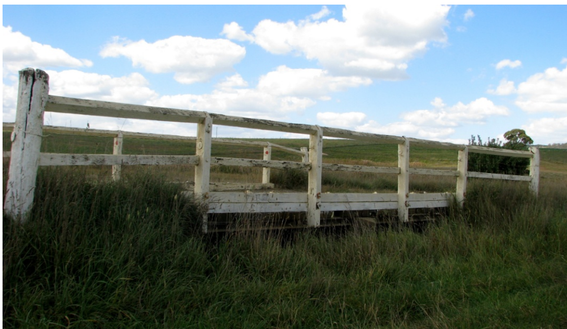
Figure 8: F30 Schumacher's Road, a timber and steel bridge
