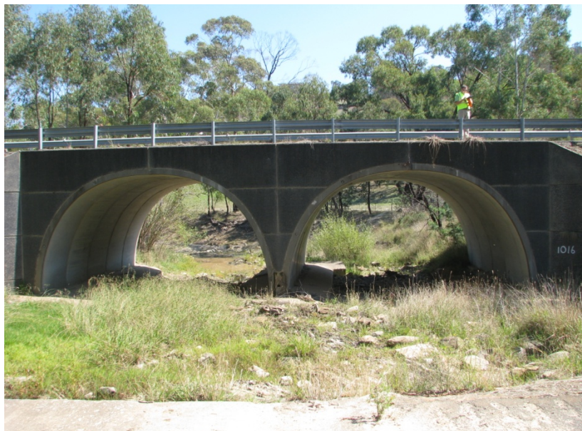
Figure 71: Large culvert technology used to form a double arched bridge on main road near Trunkey Creek (F13)
