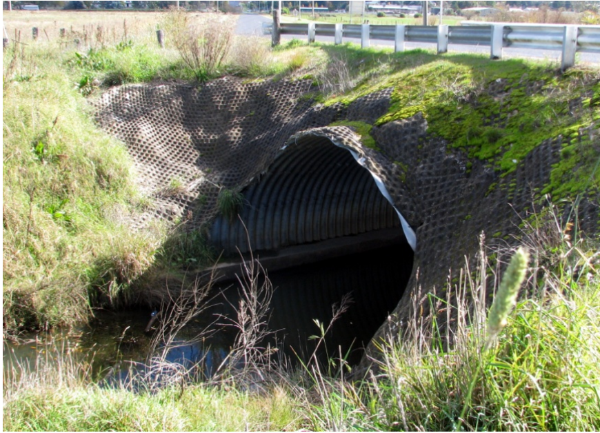
Figure 70: F57 A more recent example of the same technology with corrugated iron formed arch bridging a stream
