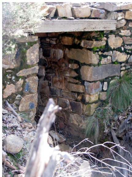
Figure 81: Cast slab over small stone bridge on the Bridle Track
