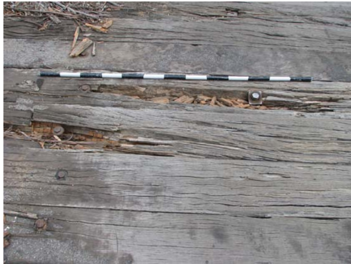
Figure 76: F83 Road deck in need of replacement above
