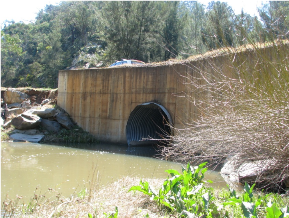
Figure 68: F21 A large pipe culvert formed from corrugated iron formwork and mass concrete on the Lachlan Road
