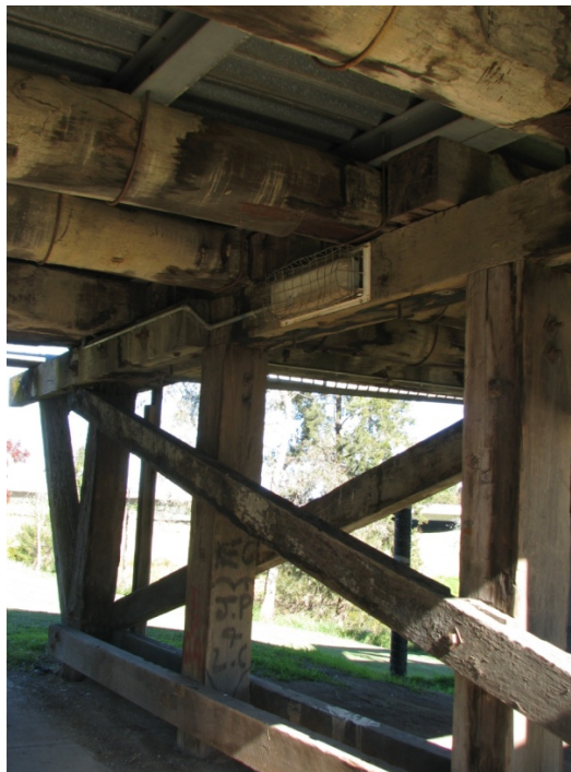
Figure 48: F64 The timber under structure of the Denison Bridge
