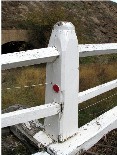
Figure 89: F85 Timber bridge post detail typical of six bridges in the LGA
