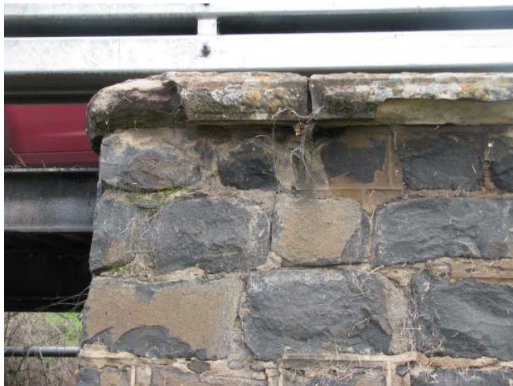
Figure 41: F141 detail in blue stone, bridge over Jordan Creek
