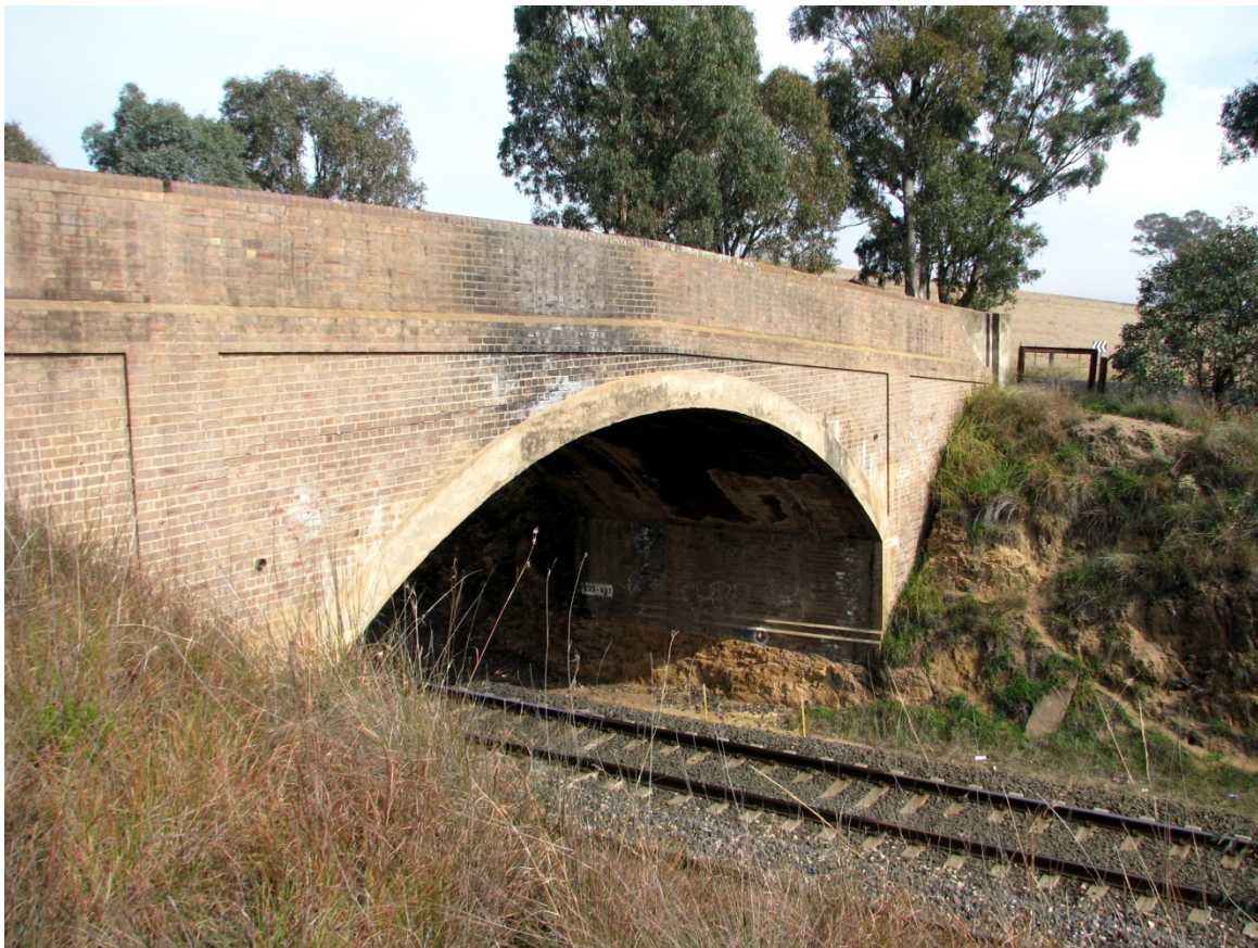
Figure 29: F73 Brewongle long single arched brick and possibly concrete bridge
