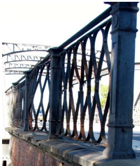
Figure 86: F59 Corroding steel balustrade on the Rocket Street bridge
