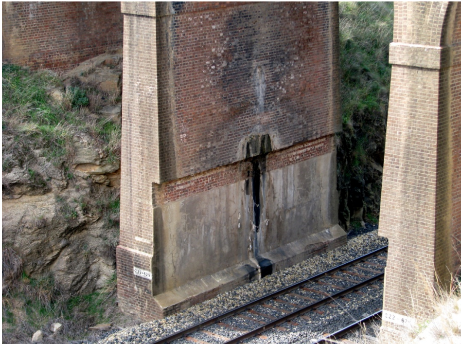
Figure 30: F74 Track side detail showing brick removal to widen the space for the second rail line
