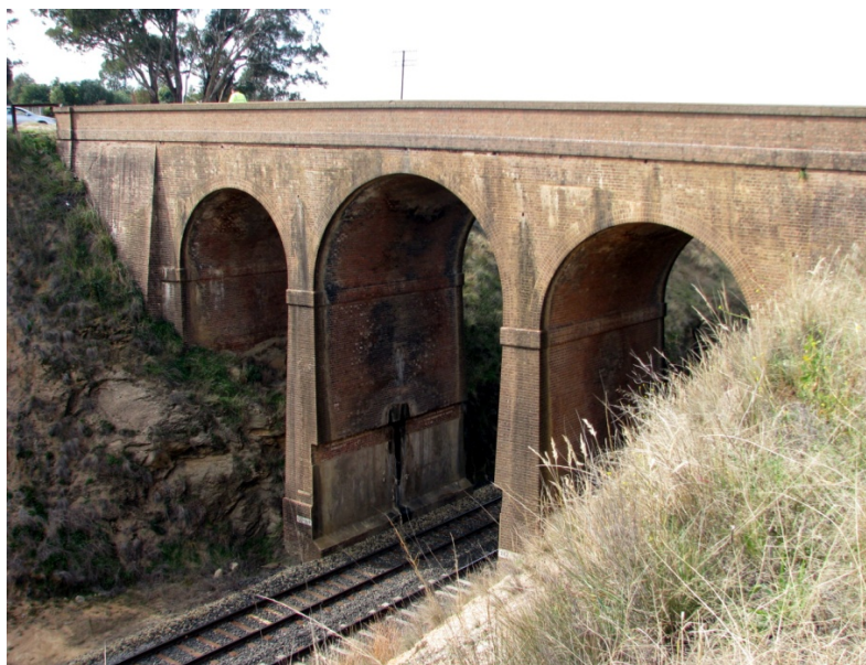
Figure 75: F74 Cracks on one side of the rail bridge are being monitored by ARTC
