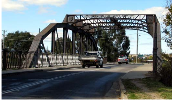
Figure 1: Rocket Street steel half through steel truss bridge
