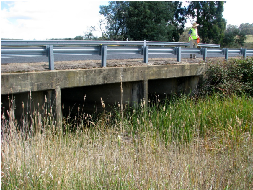
Figure 72: F28 Multiple box culvert over Buck's Creek 10 metres in width and 12 metres long
