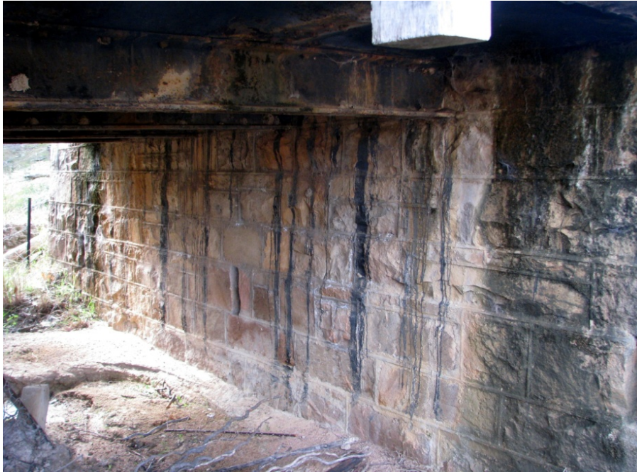
Figure 51: Sandy Creek, Ryans Road (F51) Under this stone and steel bridge 'bush' concrete material was used to seal the floor
