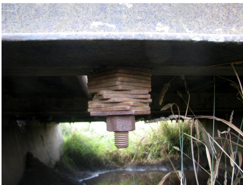
Figure 9: F30 Bolt detail below the bridge
