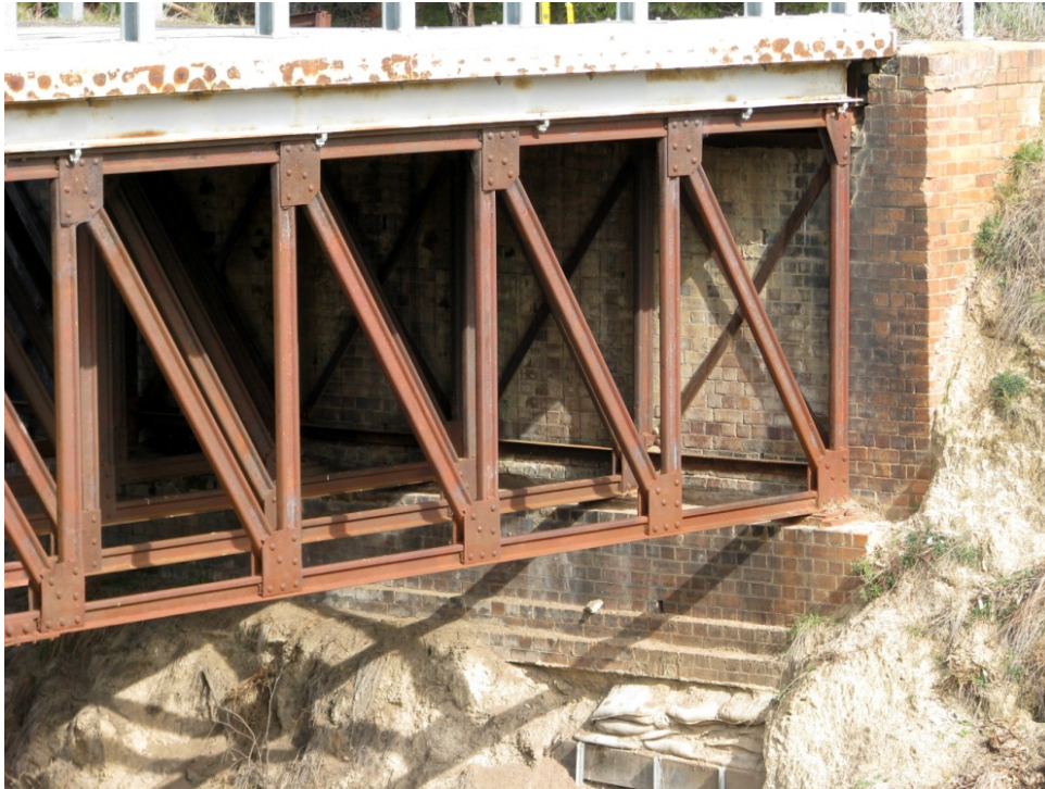
Figure 50: Detail of the 'rail line' steel sections used in the construction of the bridge (F77), using simple king post trusses
