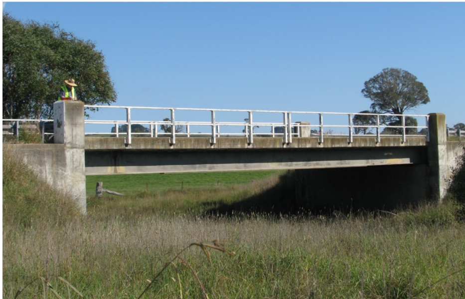
Figure 64: F20 Steel beam and concrete bridge over Caloola Creek on the Lachlan Road
