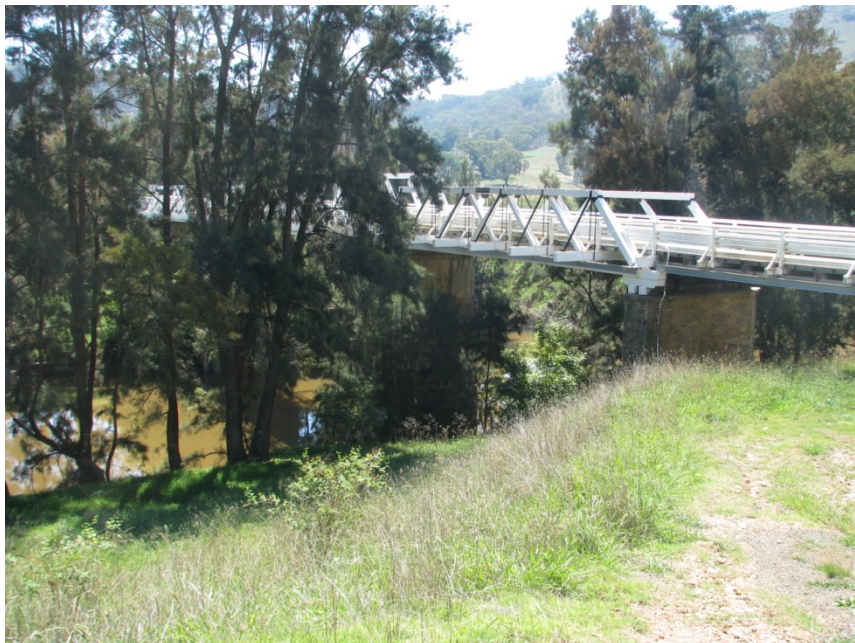
Figure 12: F12 Abercrombie River Timber Allan Truss Bridge
