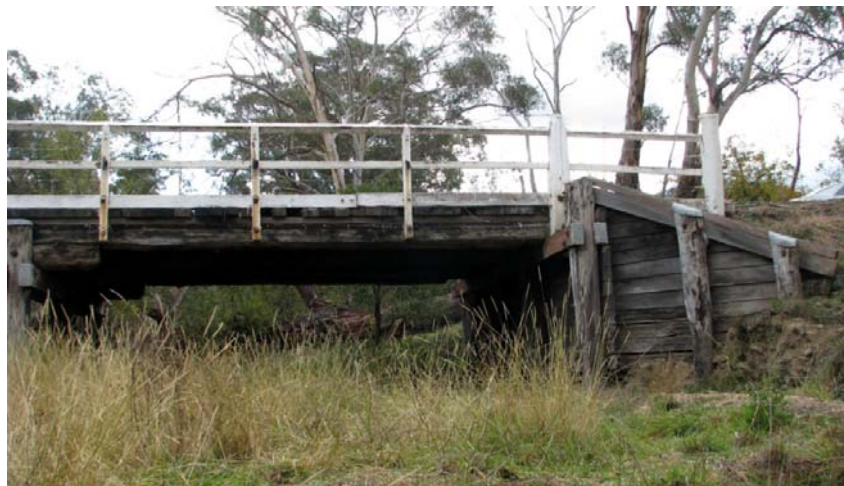
Figure 77: F83 Two span timber bridge illustrating the signs of deterioration
