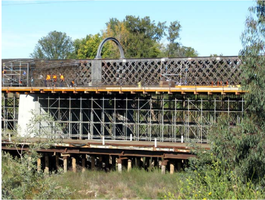
Figure 84: F63 Formwork in front of the original steel lattice bridge (20 May 2010)
