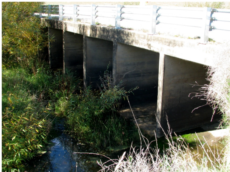
Figure 73: F37 Another multiple box culvert over Evans Creek consisting of seven box openings and an overall length of 18.5 metres, where once a considerable bridge construction would have been required.
