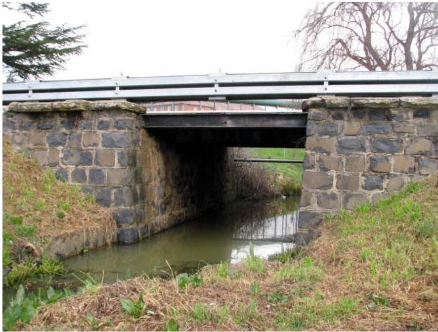
Figure 37: F141 Steel and stone ridge over Jordan Creek near Bathurst Gaol
