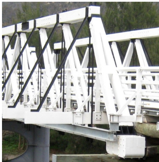
Figure 87: F144 Details of timber and steel work of the bridge over the Turon River
