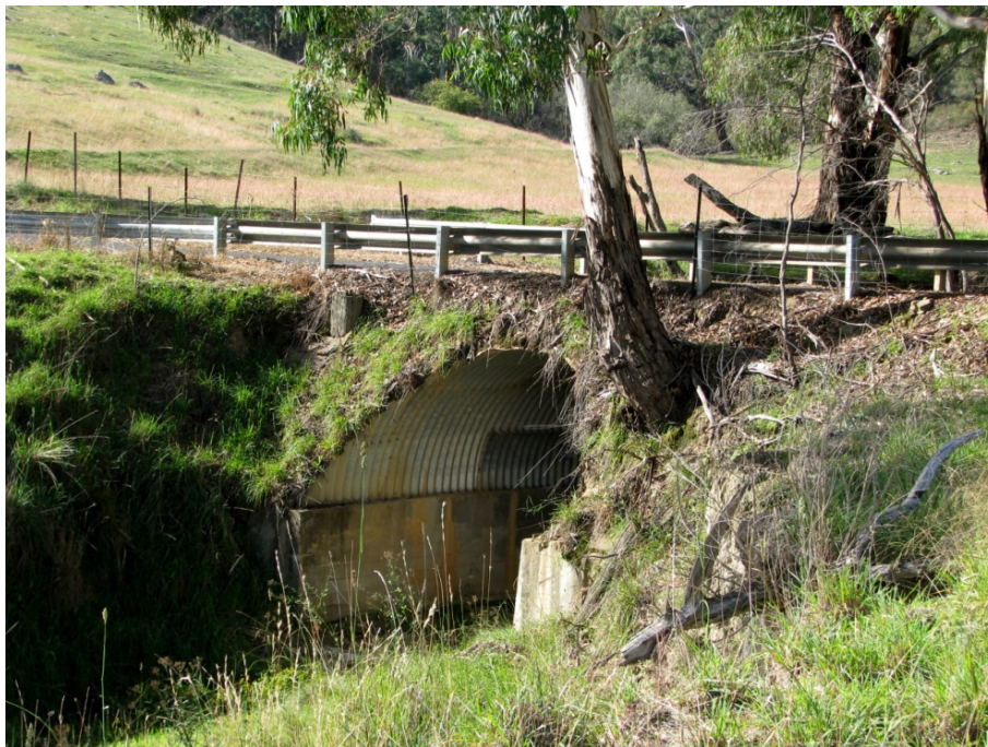
Figure 69: F46 Corrugated iron formwork is used above to form up a mass concrete arch and bridge over a stream
