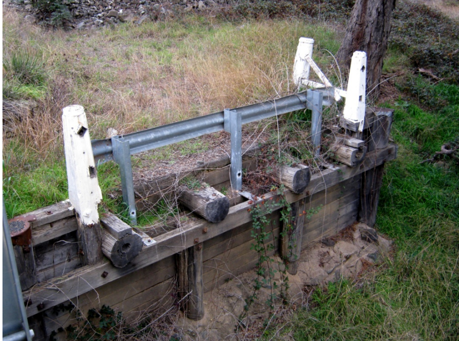
Figure 67: F123 Original timber plan abutments and shaped timber posts from a former timber bridge at Cheshire Creek
