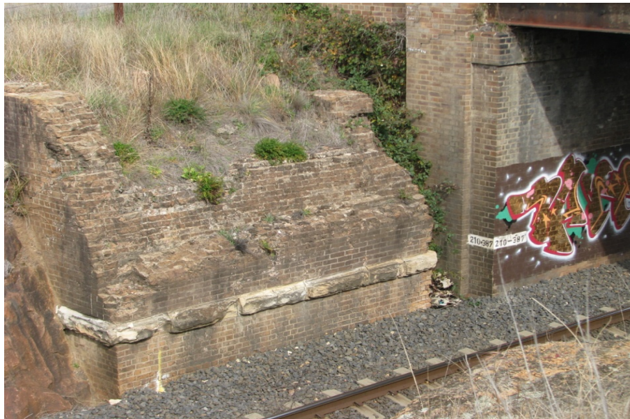
Figure 33: F82 The remains of the demolished bridge, most probably an arched brick structure
