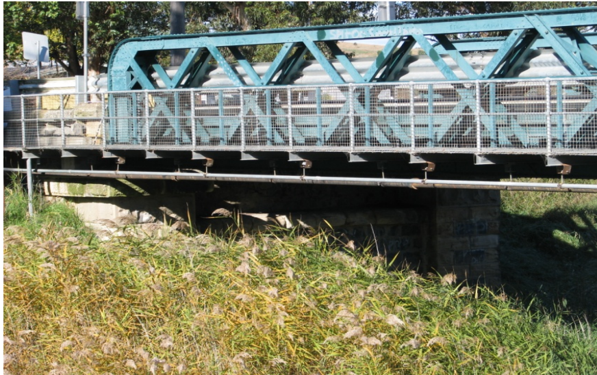
Figure 43: F49 This image illustrates the sandstone and blue stone abutments
