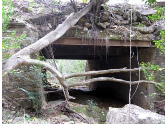
Figure 78: F118 This steel and stone bridge is now well below road level and difficult to inspect
