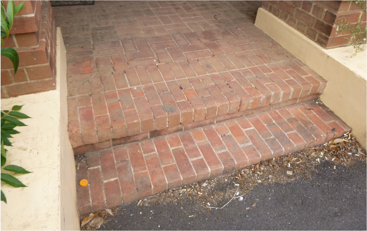
Figure 35 View of the vestibule area including entry stairs.
