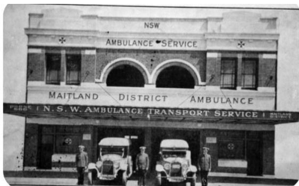
Figure 44 Maitland Ambulance Station. Source: Flickr.
