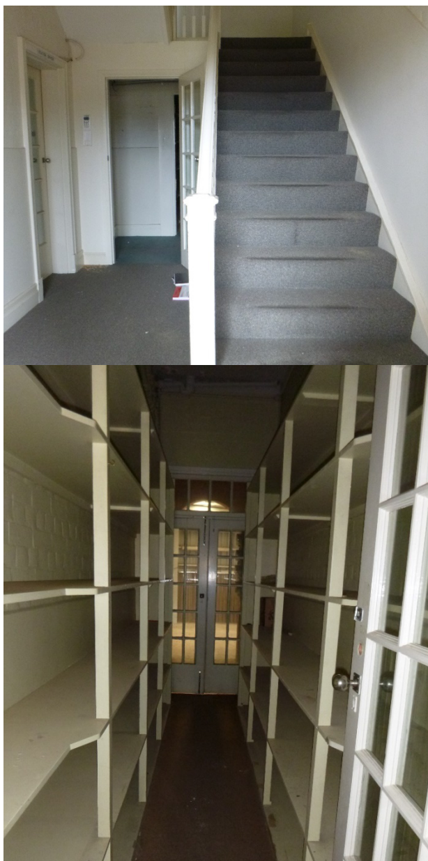
Figure 34 Entry stairs and passage between ambulance bays leading to the rear yard.
