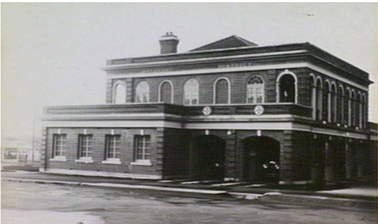
Figure 21 Undated Post card (prior to 1941) of the Bathurst District Ambulance Station held in the State Library of Victoria. Source: SLVIC image a09760
