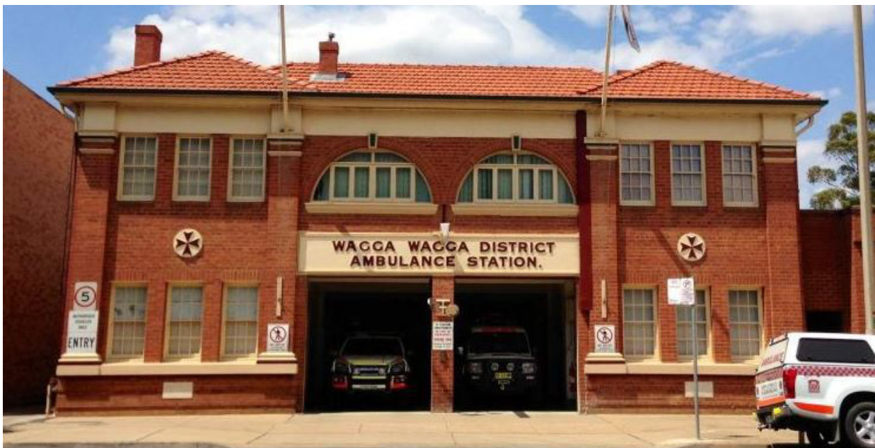
Figure 45 Wagga Wagga Ambulance Station
