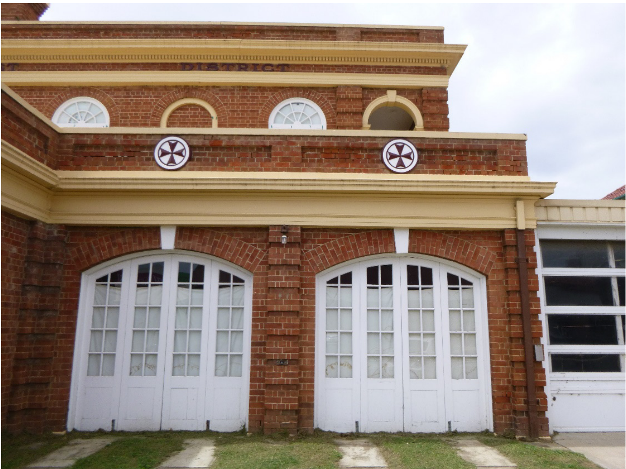
Figure 29 View of the Ambulance Bay Doors, Bathurst District Ambulance Station.
