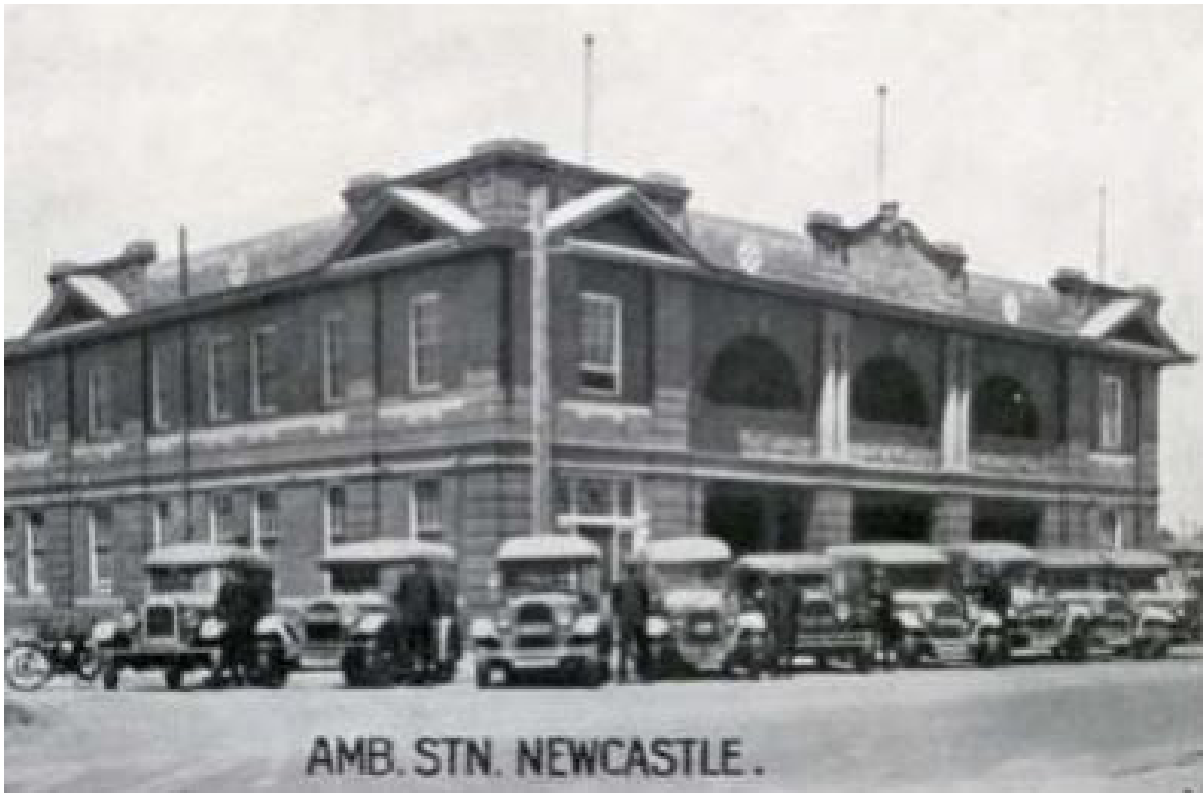
Figure 43 Ambulance Station, Newcastle. Source: Flickr.
