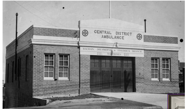
Figure 42 Drummoyne Ambulance Station (demolished)
