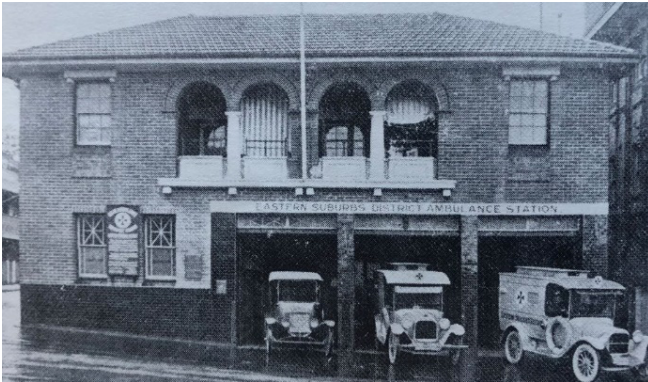
Figure 41 Coogee Ambulance Station (much altered)
