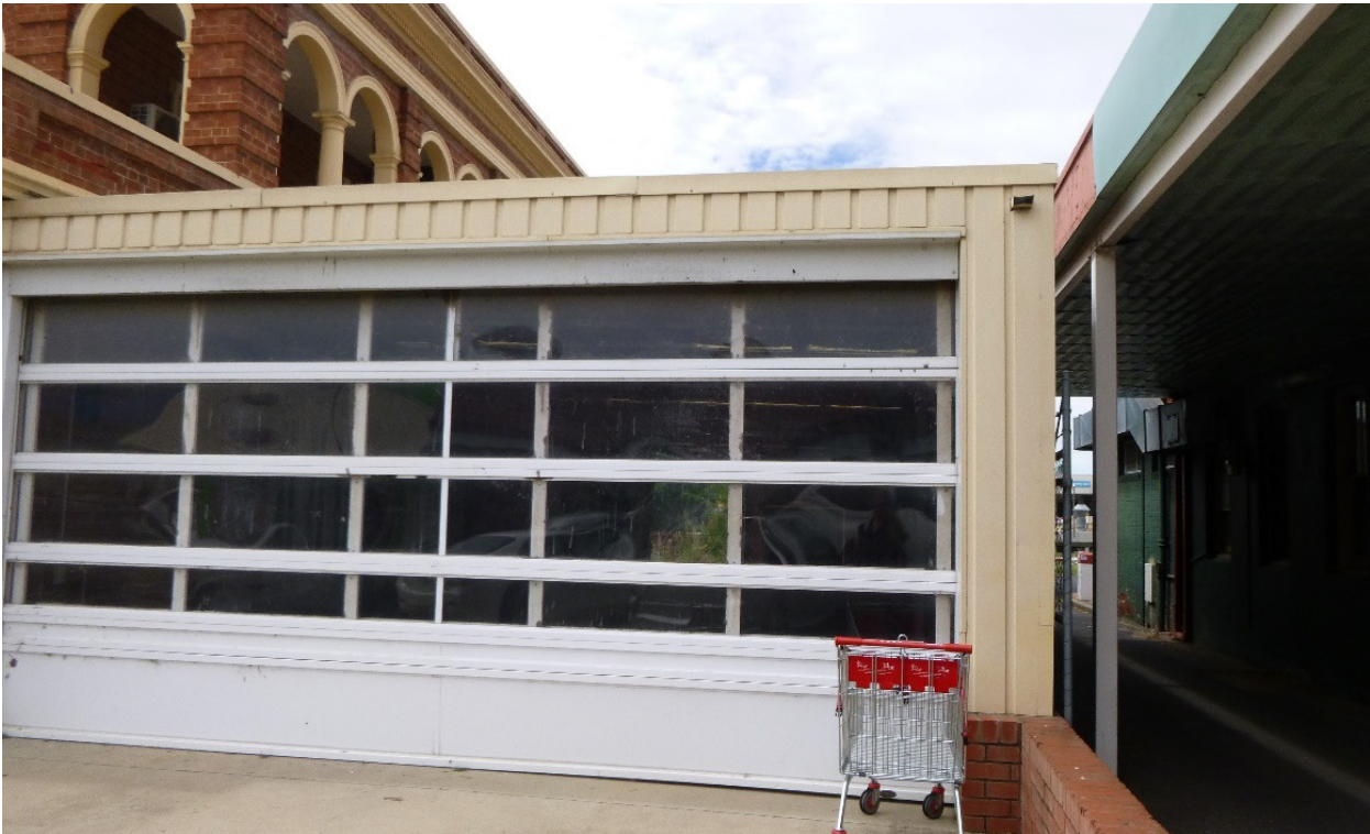
Figure 30 View of the modern covered area, Bathurst District Ambulance Station.
