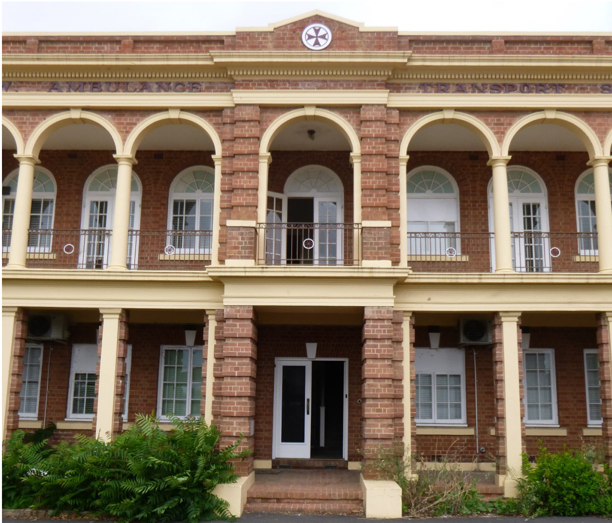
Figure 25 Main entrance located in the façade facing the reserve, showing the logo and station name on the brick frieze, below the pediment bearing the Ambulance Service logo.
