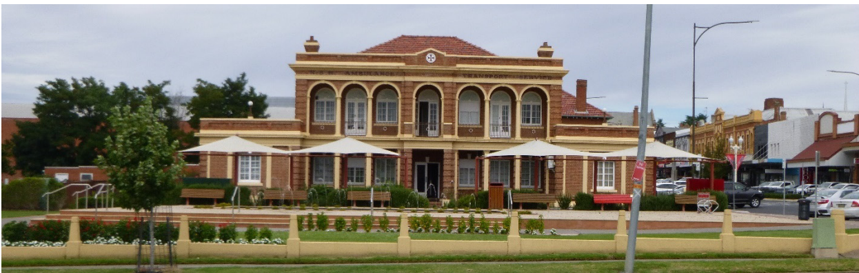
Figure 22 View of the main front of the former Bathurst District Ambulance Station.
