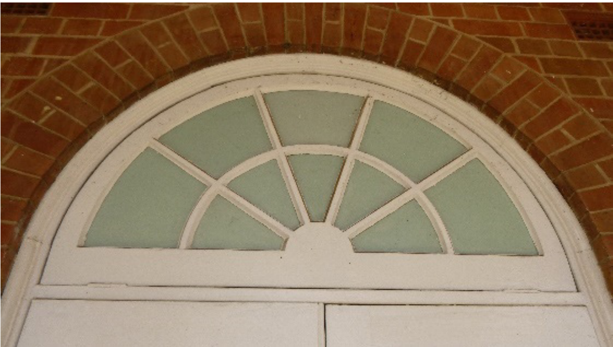
Figure 27 Fanlight over French doors onto terrace area on first floor.
