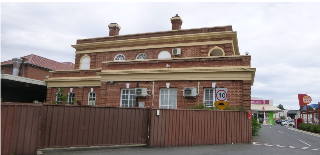
Figure 31 Side View of the Bathurst District Ambulance Station.
