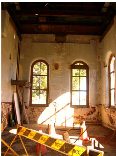
Figure 15 Pump room from north showing evidence of original dado
