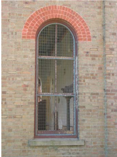
Figure 4 Original window. The centre sash of these windows was a pivot.
