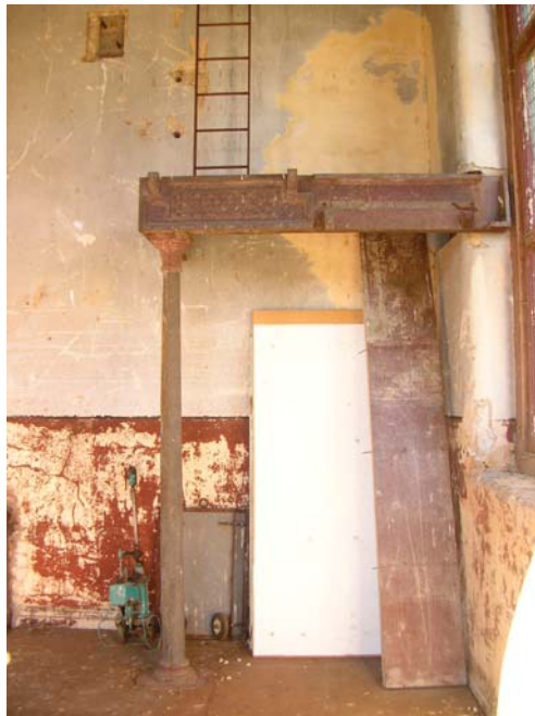
Figure 17 Original cast iron platform in southeast corner of pump room.
