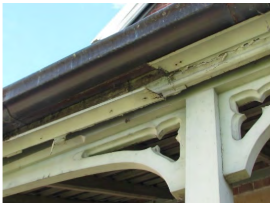
Figure 9 Part 6: Deteriorating eaves detail Block C
