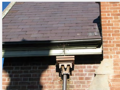
Figure 12 Part 4: Gutters and downpipes generally need reseating
