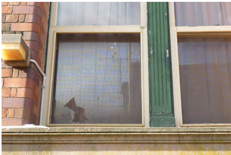
Figure 3 Part 6: Cracked window glass, flaking window paint. The light fitting on the right hand side if no longer used should be removed
