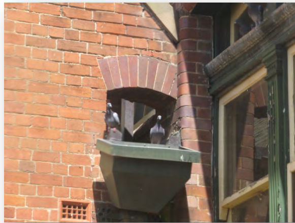
Figure 3 Part 10: The rainwater head falling away from the building. While making this repair an opportunity will be there to check the roof plumbing generally and report back
