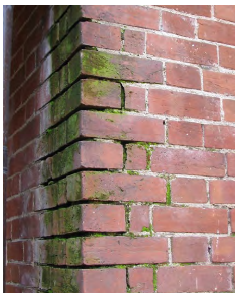
Figure 4 Part 6: Eroded mortar joints and unsightly moss growth which requires cleaning and repointing
