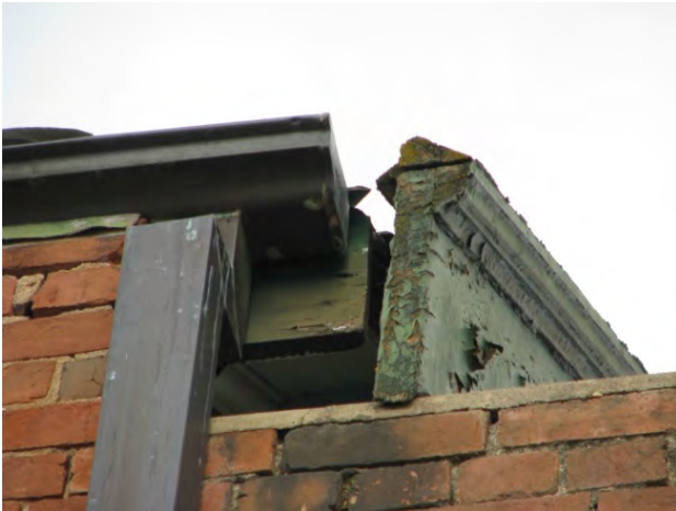
Figure 3 Part 8: Deteriorated junction of gable end above caretaker's flat
