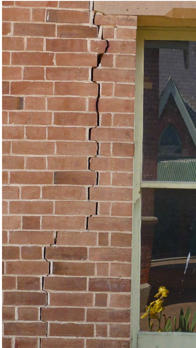
Figure 1 Part 6: Cracked wall in former Headmaster's residence
