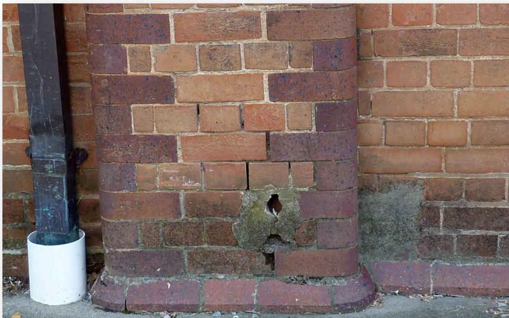
Figure 2: Poorly executed repairs and paint downpipe base
