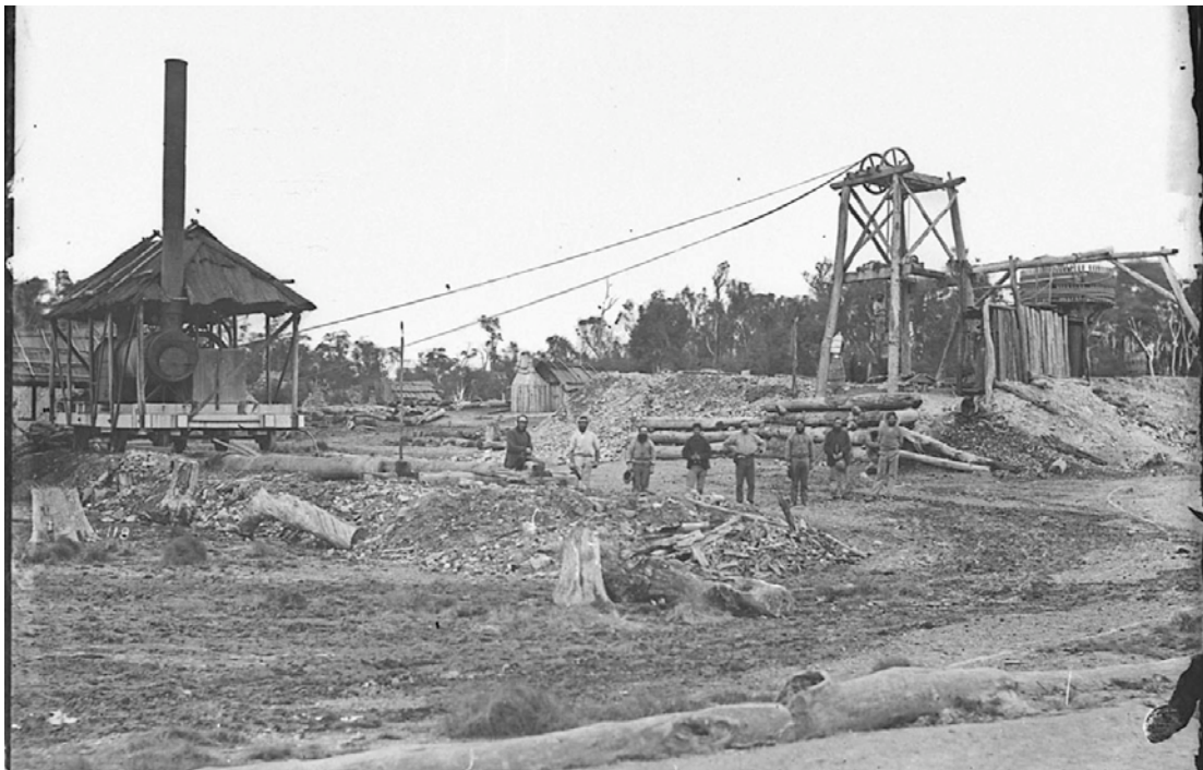
Figure 9.6. A general view of the goldmine at Wilson's Reef, Trunkey, showing a donkey steam engine on rails, powering the poppet head and a whim.
