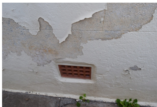
Figure 81 Plaster peeling on the external wall on the east side of the cottage
