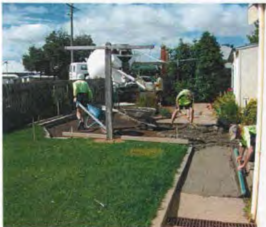
Image 2: Pouring and laying new concrete at Chifley Home
