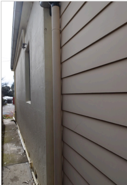
Figure 125 Western wall—new construction in weatherboard is evident
