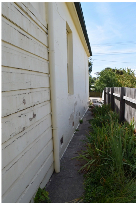
Figure 82 Eastern façade—paint peeling is evident, but not severe.
