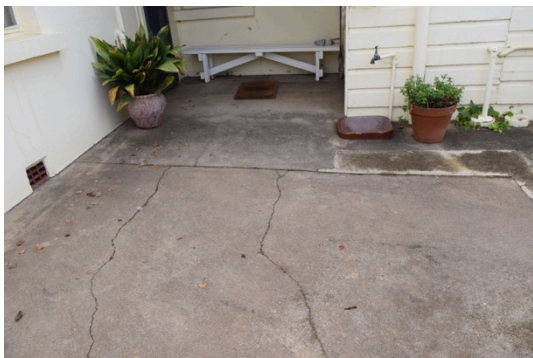
Figure 95 External concreted area (rear verandah)—note the cracks on the concreting (this section was identified in 2010 as not original to the Chifley period – Appendix 4)
