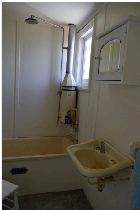
Figure 63 Bathroom—enclosed from a section of the rear verandah. Hot water mechanism for shower and sink.
