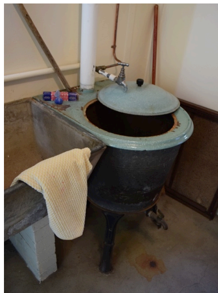
Figure 68 Gas-heated boiler
