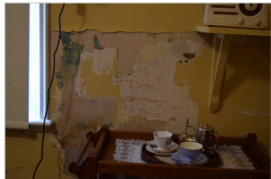
Figure 58 Damage to the plaster of the external wall is clearly evident.
