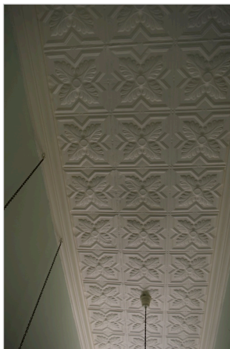
Figure 44 Pressed metal ceiling detail in the hallway
