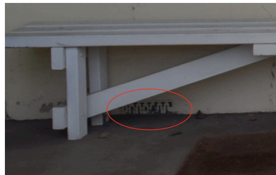
Figure 96 External concreted area (rear verandah)—note the partially concealed vent below the seat (indicated).
