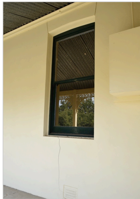
Figure 122 Front window along the verandah—note the crack below the window sill
