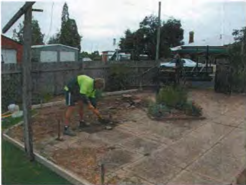
Image 1: Removing damaged concrete at Chifley Home
