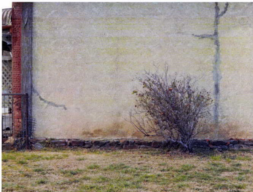
Plate 6: Stone footings and wall cracking
