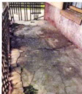
Verandah floor cracking
