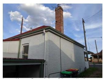
Image 18 General view of the rear North west corner of the cottage noting the simple four room bulk which sits beneath the hipped roof with the timber framed rear skillion to the rear.
