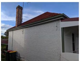
Image 16 A general view of the West Elevation, noting the wall tie rods, damaged chimney brickwork and the metal roof – 'Decramastic' tile sheeting provided to emulate a tile roof.
