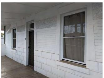
Image 13 The ashlar cement rendered dado wall treatment, inter-war inclined window surrounds to the aluminium double hung sliding sash and roughcast panels to the front facade.
