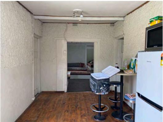
**Plate 3.13:** Area created by enclosure of the northern courtyard in the late 20<sup>th</sup> century. The original back door of the bungalow is in the centre and doorways to 1920s wing extensions on each side.
