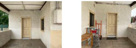
Plates 3.3 & 3.4: The western & eastern sleeping porches. The concrete floor of the porch areas is in fair to poor condition. Note new aluminium windows on either side of the living room. The doors do not appear to be original.
