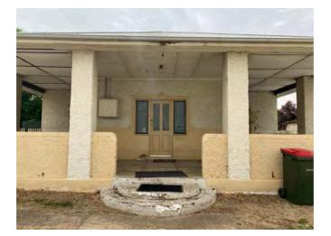
Plate 3.2: The central entry porch showing semi-circular front steps, columns and front door with sidelights. Note the simple rendered bracketing around the doorway. The panelled ceiling is lined with plaster sheets. This suggests a construction date prior to 1917, the year of commencement of manufacture of fibrolite sheeting in Australia.
