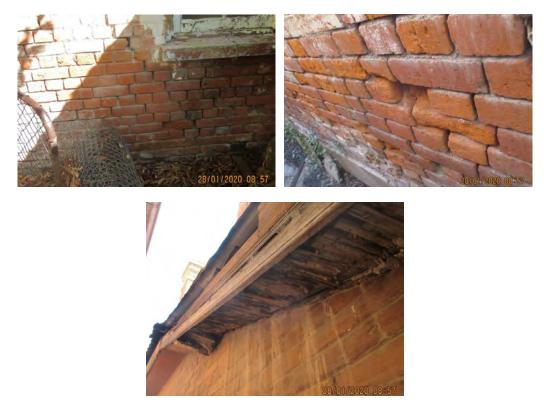
External timber (structural and non-structural) and eaves material displayed extreme weather damage at the time of our inspection.
