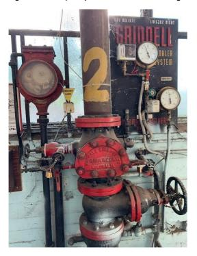
Figure 3: fire sprinkler system valve set
