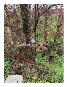
Figure 1: Booster assembly on Browning Street
