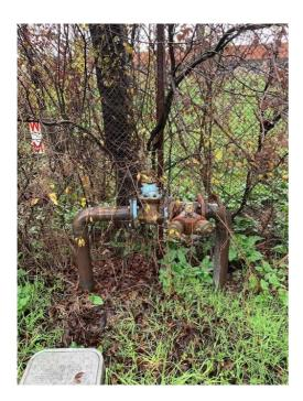
Figure 1: Booster assembly on Browning Street
