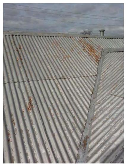
Roof sheets are loose in various places and should be screwed down.
