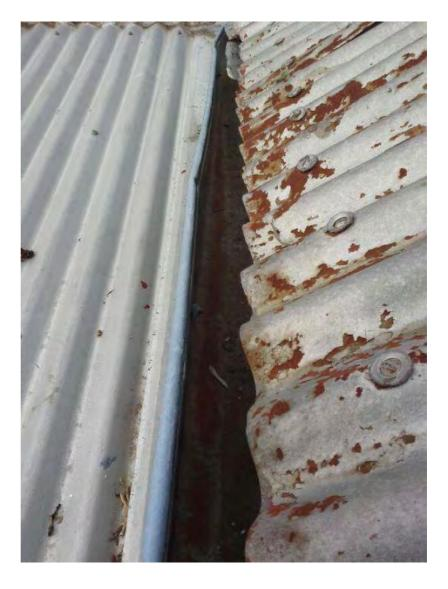
The stop end is missing to the front gutter. This should be installed.
