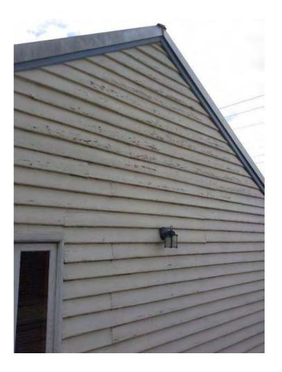
Minor fine cracks are visible. These appear to be caused by a little typical expansion and contraction.
