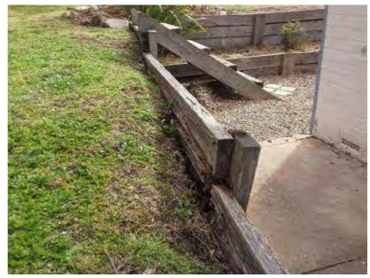
The hardwood timber retaining walls/garden edging show normal deterioration and decay. These timbers should be replaced with durable materials.
