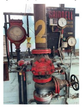
Figure 3: fire sprinkler system valve set
