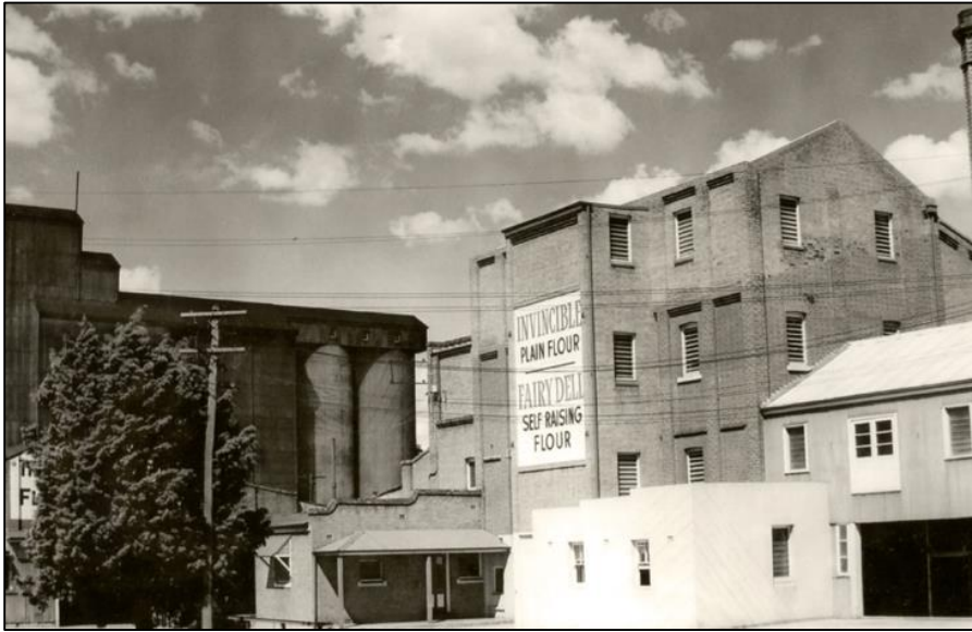
Figure 53: View of mill, 1970s.
