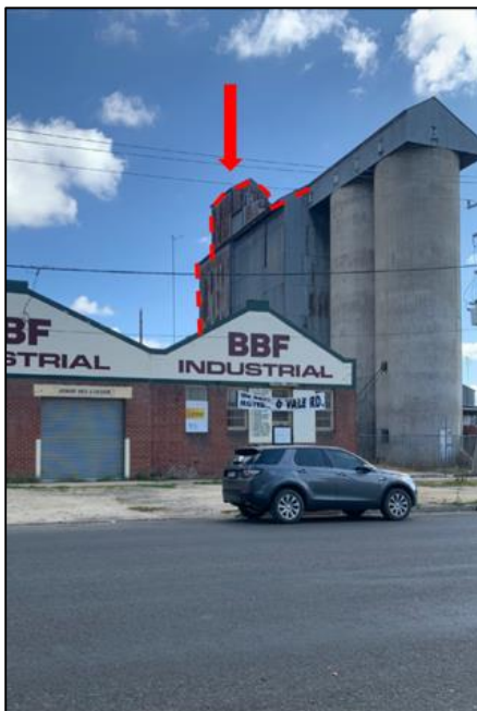
Figure 65: Timber silos as viewed from Havannah Street.
