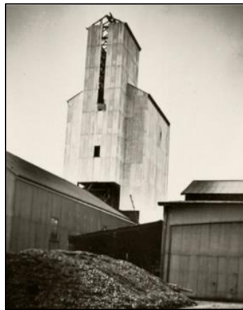
Figure 45: Nine-bin silo, 1932. Tremain Family Archives
