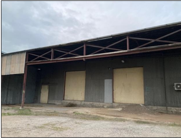
Figure 72: Weighbridge and Siding as viewed from within the site.
