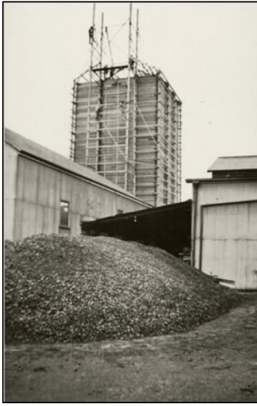
Figure 35: Large shed (right) and smaller shed (left), 1932. Tremain Family Archives
