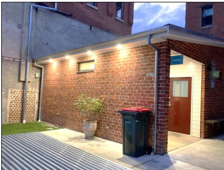
Figure 69: The Amenities Block as viewed within the site.
