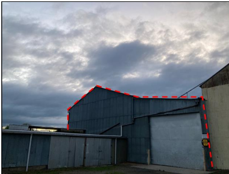
Figure 73: Bedwells Rear Warehouse as viewed from Manilla Street.
