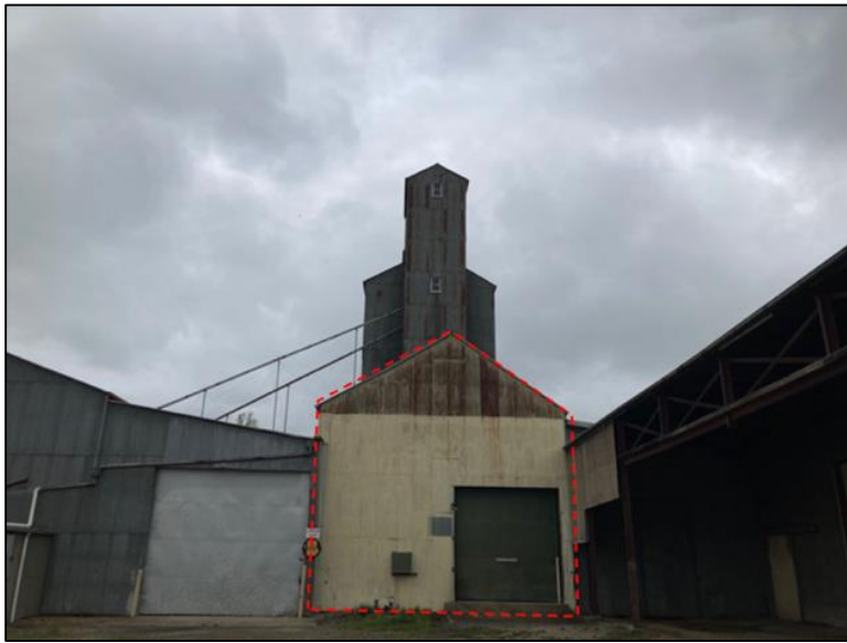
Figure 64: Building 11 viewed from Manilla Street.
