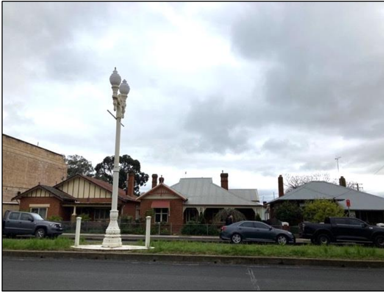
Figure 79: An example of single-storey Federation period cottages to the north of the site.
