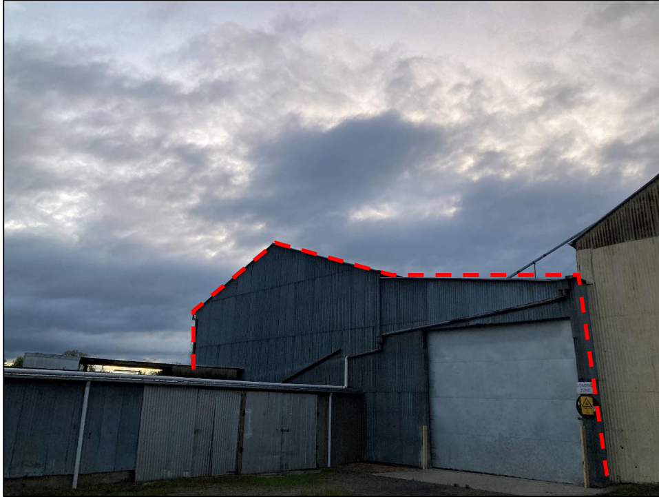
Figure 20: Bedwells Rear Warehouse as viewed from Manilla Street.
