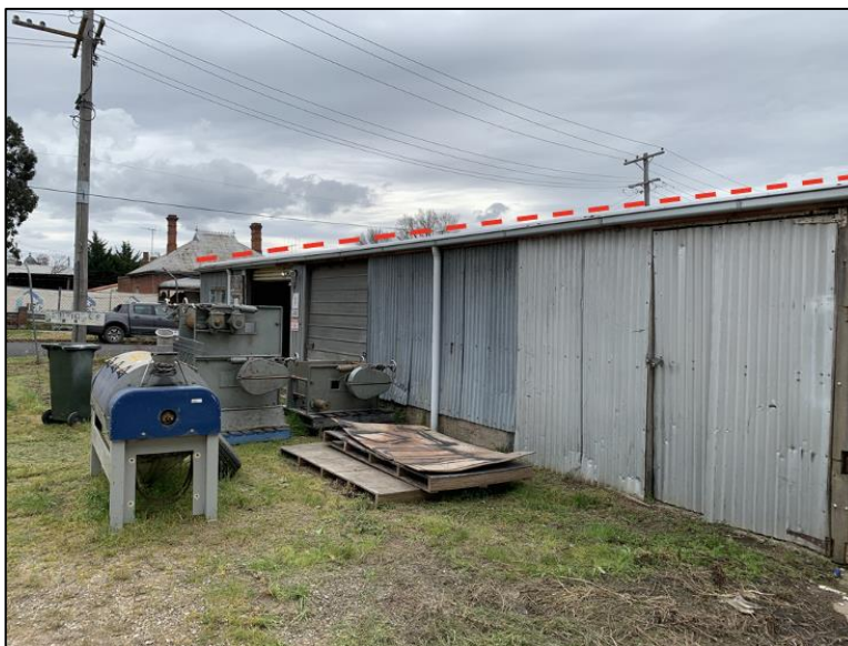
Figure 75: The garages as viewed from within the site near Manilla Street.
