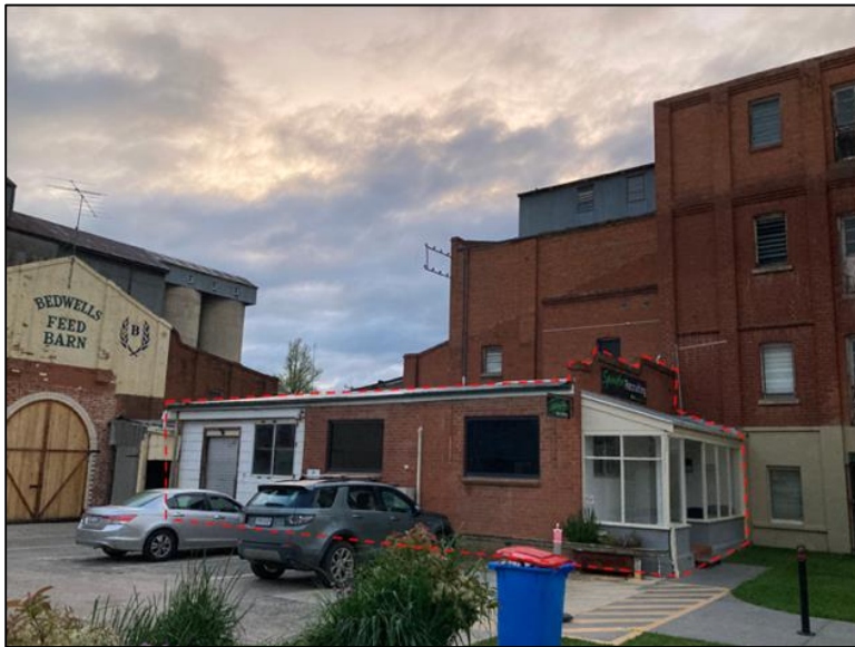
Figure 70: The Mill Office as viewed within the site.
