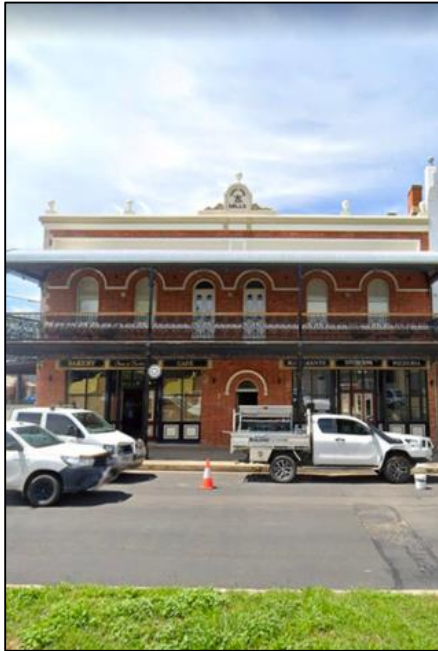
Figure 60: Victoria Stores Building as viewed from Keppel Street.
