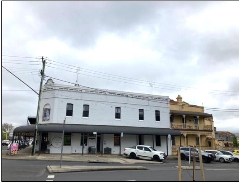
Figure 77: No. 3 Keppel Street to the south of the site.
