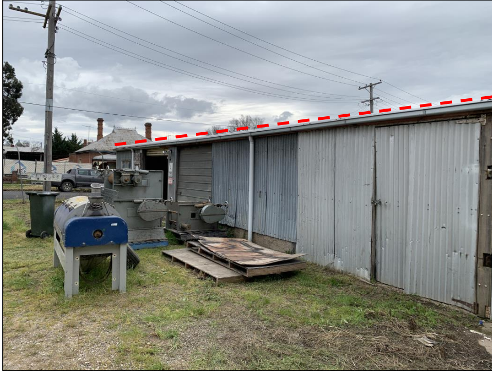
Figure 22: Garages as viewed from within the site near Manilla Street.
