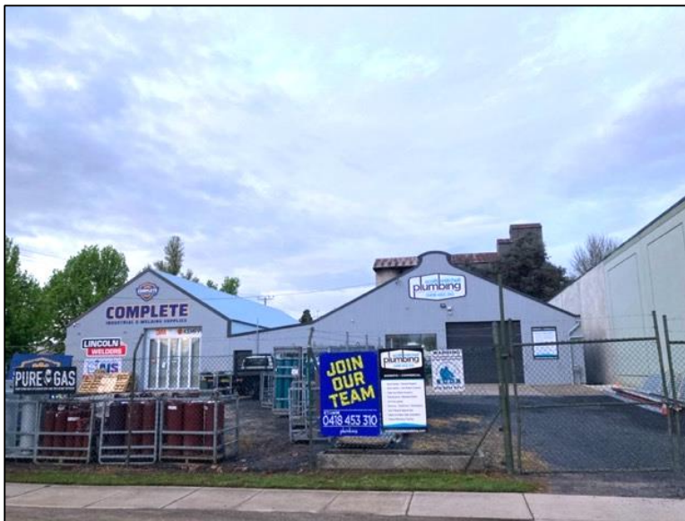
Figure 84: An example of 20 th century period commercial buildings on the north side of Havannah Street, to the east of the site.
