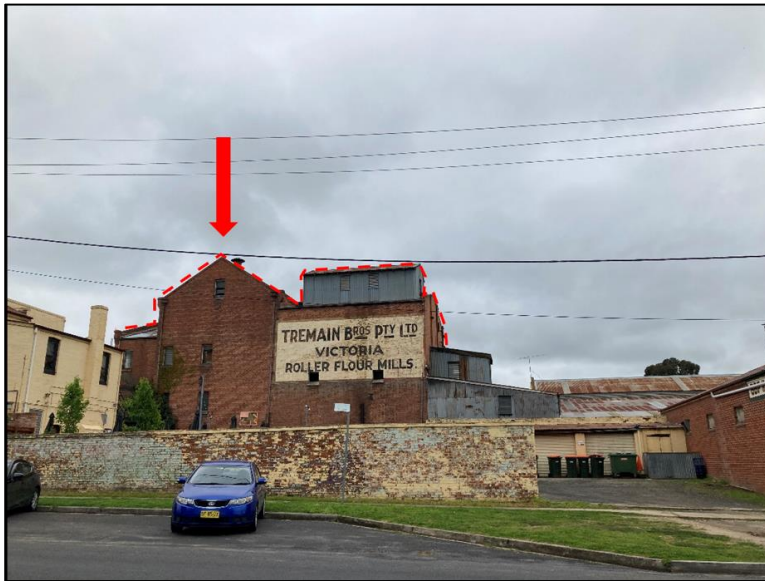
Figure 62: The rear of the Mill Building viewed from Havannah Street. The corrugated iron structure on the roof is visible above the Tremain logo.
