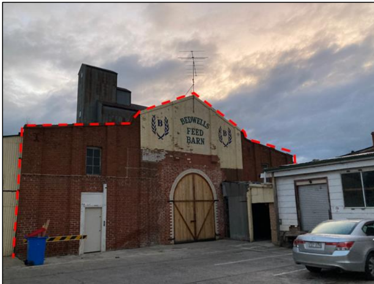
Figure 63: Bedwells Feed Barn Warehouse as viewed within the site.
