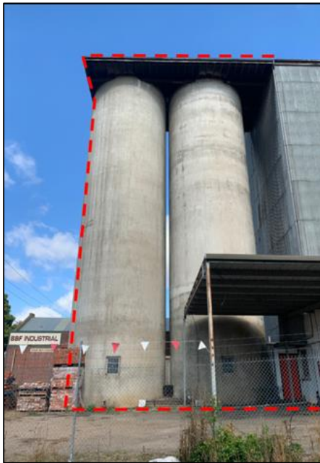
Figure 66: Concrete silos as viewed from within the site.
