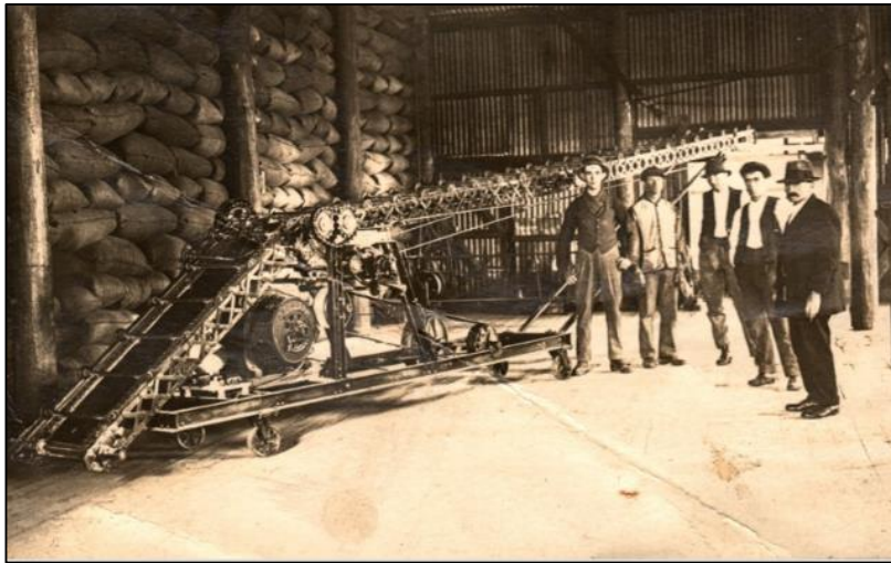
Figure 33: Electric bag elevator, 1918. Tremain Family Archives
