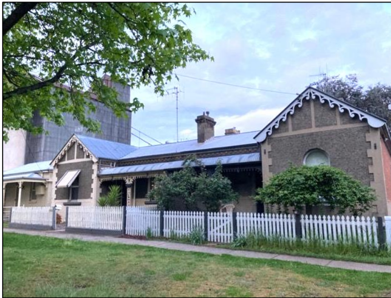
Figure 82: An example of Victorian period cottages to the east of the site on the north side of Havannah Street.
