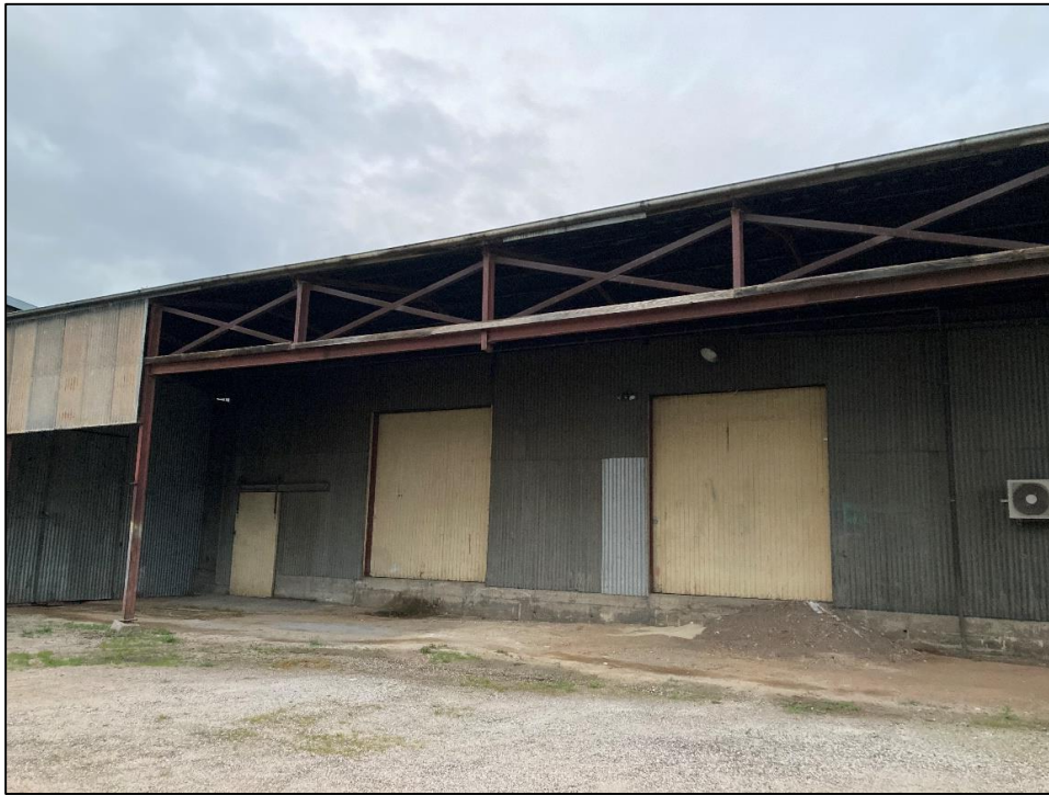
Figure 19: Weighbridge and Siding as viewed within the site.
