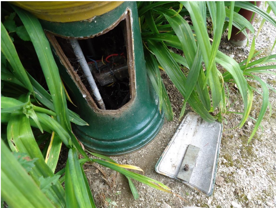
Photo 39: Replaced galvanised anchor and galvanised access plate
