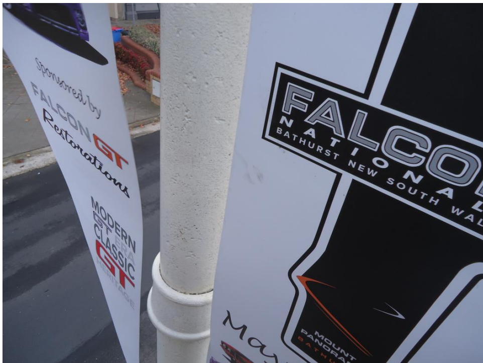
Photo 18: Pitting in post, further corrosion prevented from quality paint coating (note some defects may be from initial casting)
