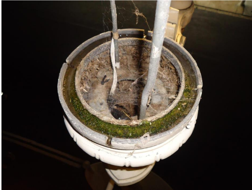
Photo 1: Build up of lichen and moss in the Lamp Base
