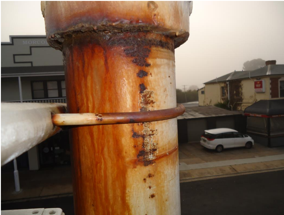
Photo 23: Corrosion at component junctions
