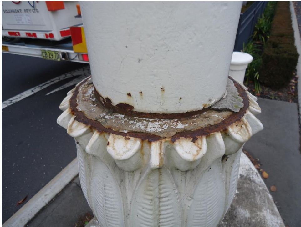
Photo 17: Grout seal in poor condition
