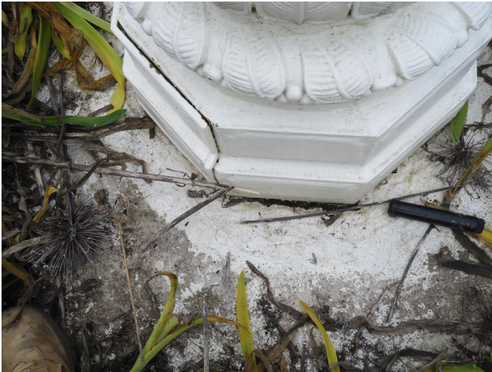
Photo 29: Poor sealing of Base against concrete
