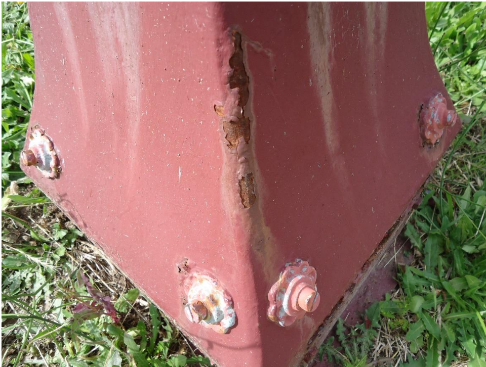
Photo 48: Corrosion showing through external paint
