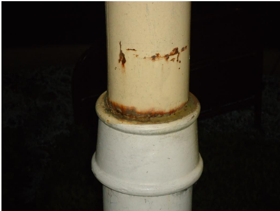
Photo 20: Mastic sealant between collar and post at the end of its life
