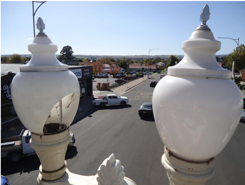
Photo 12: Broken Globe permitting water ingress and access for insects
