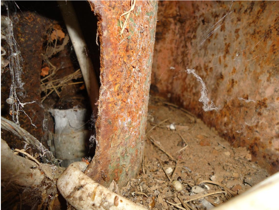
Photo 49: Corrosion of cast in post
