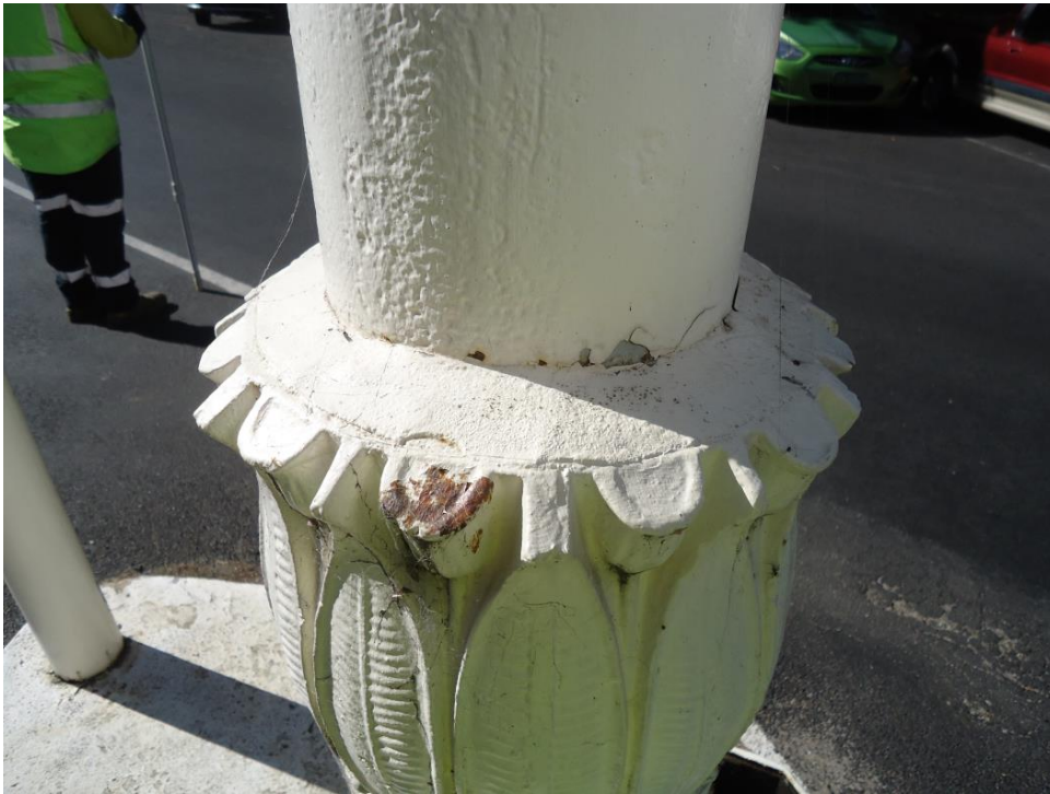
Photo 15: Grout seal in good condition
