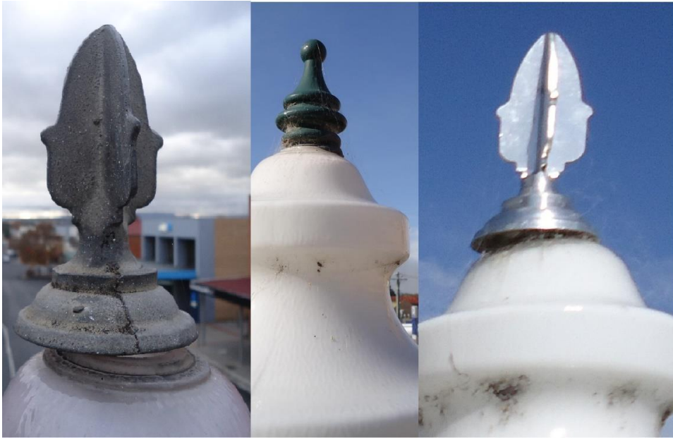
Photo 7: Variation in Finial design, original on left, older replacement in centre and recent replica on right
