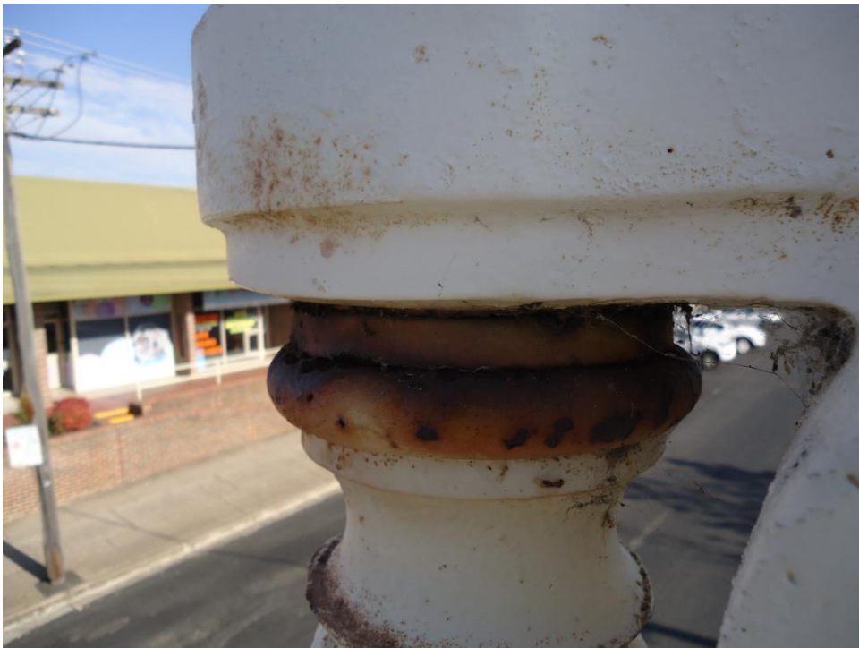
Photo 24: Corrosion at Base Finial and Centre Moulding
