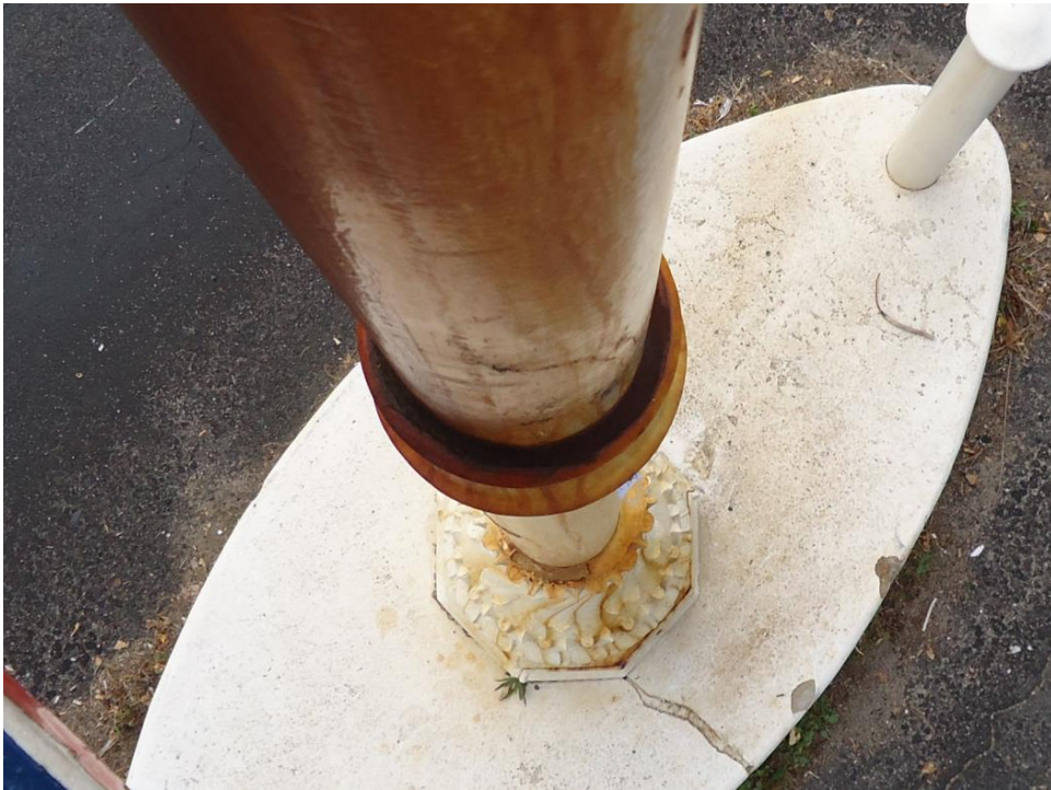
Photo 21: Corrosion from water ingress in collar
