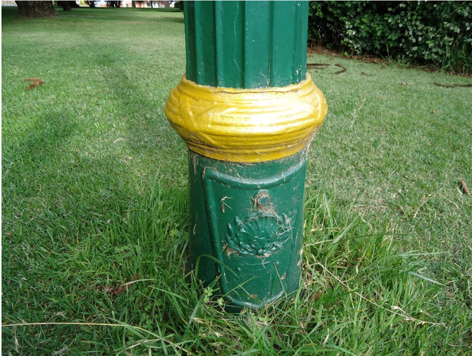
Photo 40: Original Base and Access Plate with good condition paint
