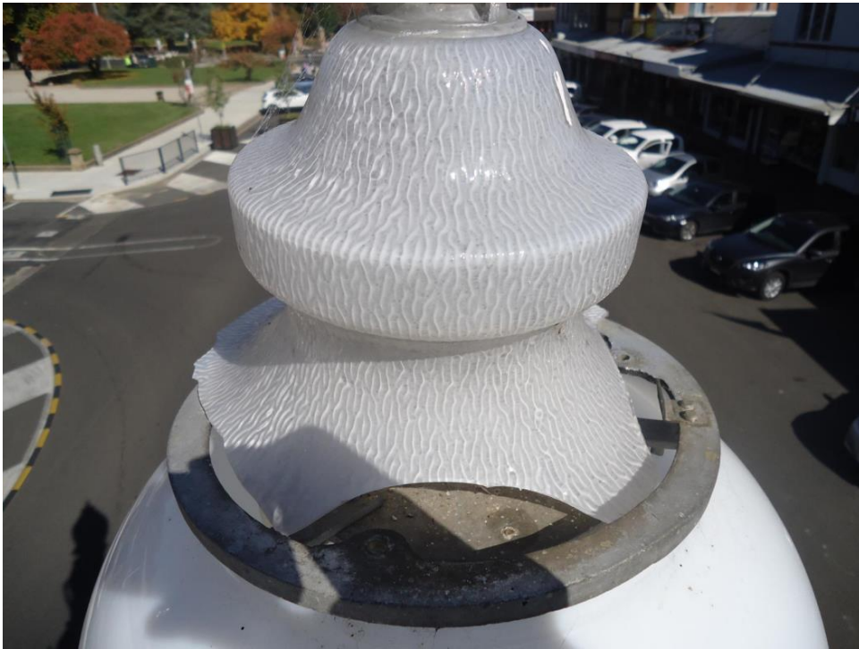
Photo 11: Broken Canopy permitting water ingress and access for insects
