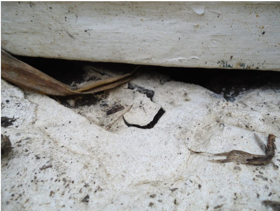
Photo 30: Close-up of poor Base/concrete seal
