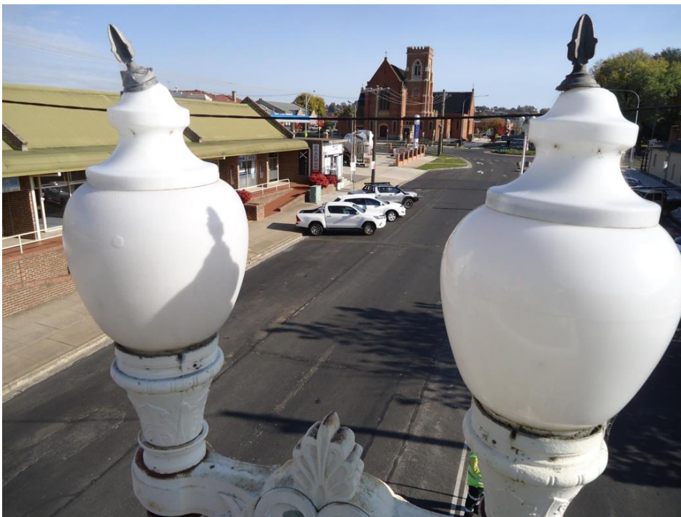
Photo 8: Skewed Finials and retaining rod resulting in poor seal and permitting water ingress and access for insects
