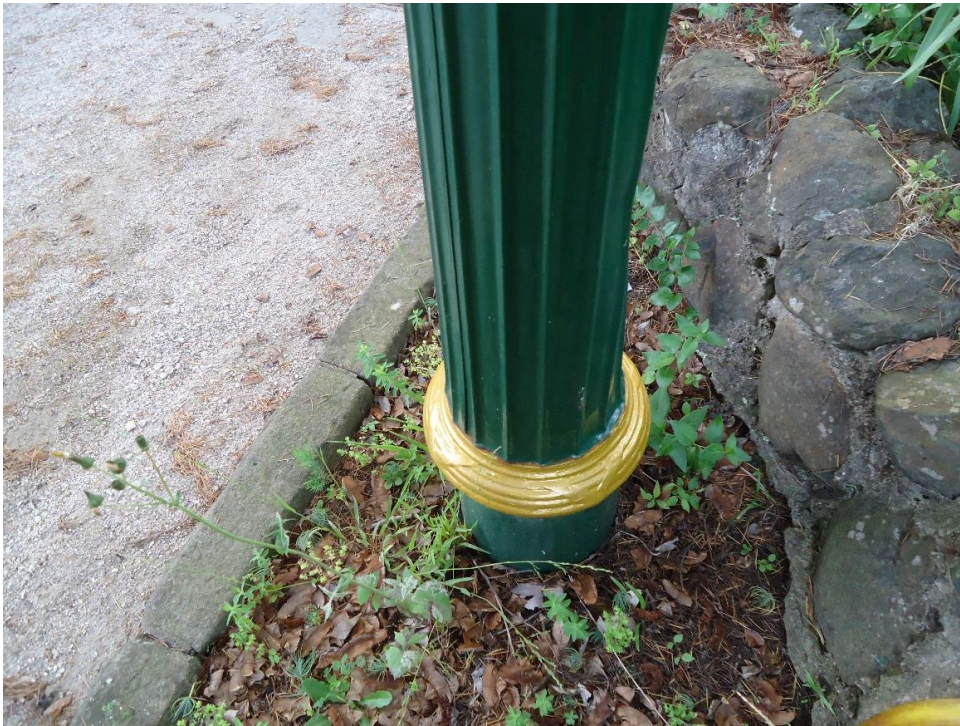
Photo 42: Buried lamp bases accelerating corrosion
