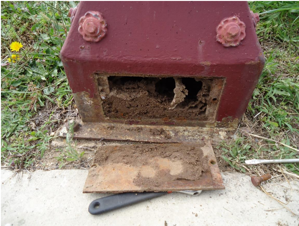
Photo 46: Excessive build up of dirt contributing to corrosion
