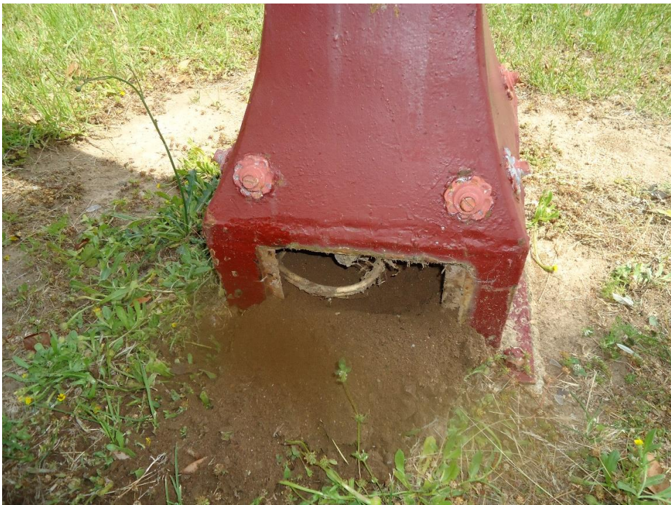
Photo 45: Excessive build up of dirt contributing to corrosion
