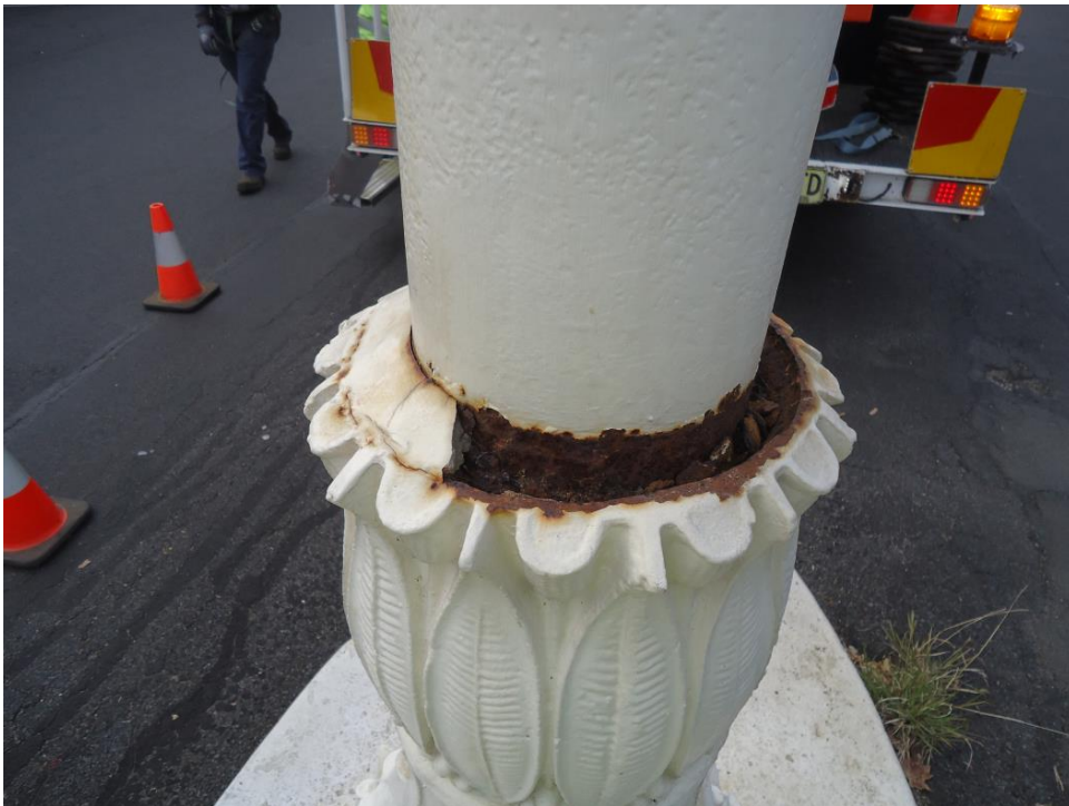
Photo 16: Grout Seal in very poor condition
