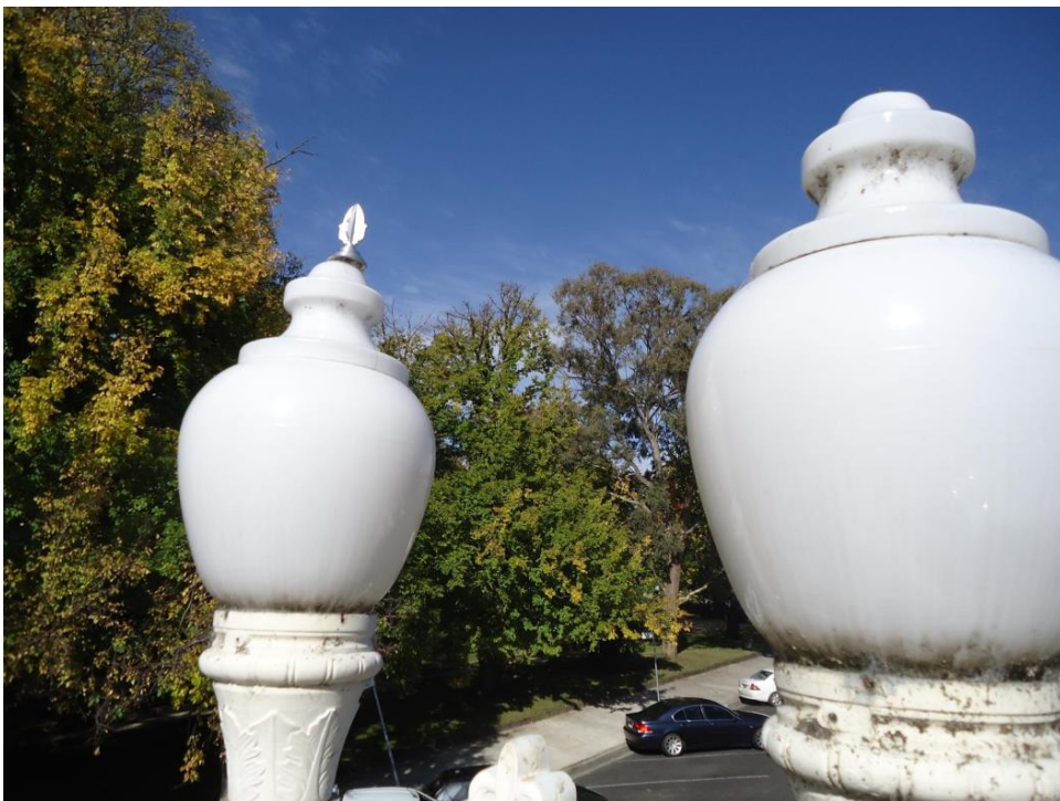
Photo 10: Skewed and missing Finials resulting in poor seal and permitting water ingress and access for insects
