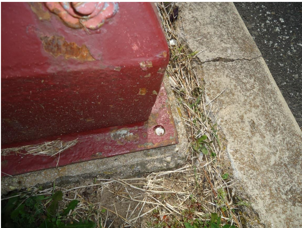
Photo 54: Ineffective fastener on same lamp as Photo 52 and Photo 53
