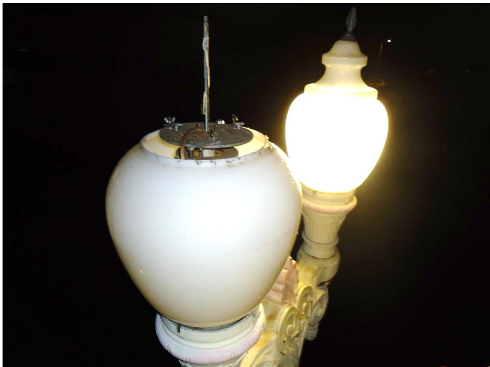
Photo 4: Finial and Canopy retaining rod
