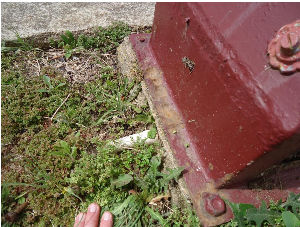
Photo 52: Ineffective fastener top of photo
