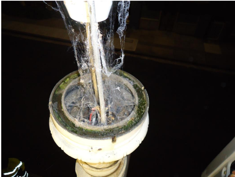
Photo 3: Build up of lichen and moss in the Lamp Base
