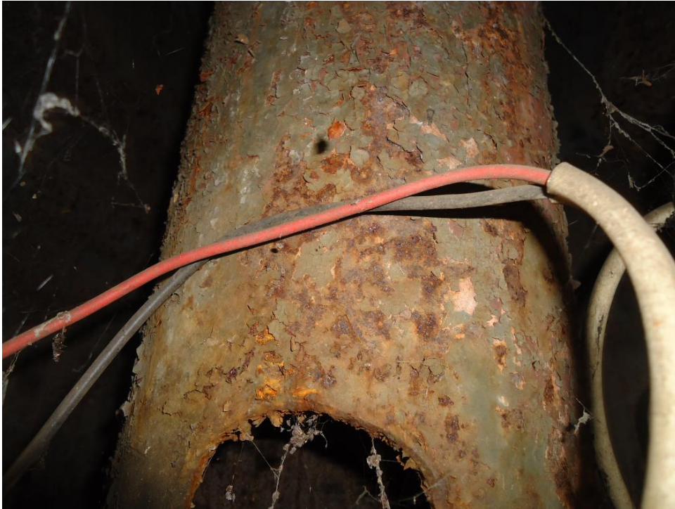
Photo 27: Surface corrosion at base of the Post
