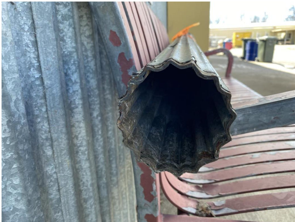
Photo 33: Top of galvanised rolled post – Machattie Park and Kings Parade Lamp Standard
