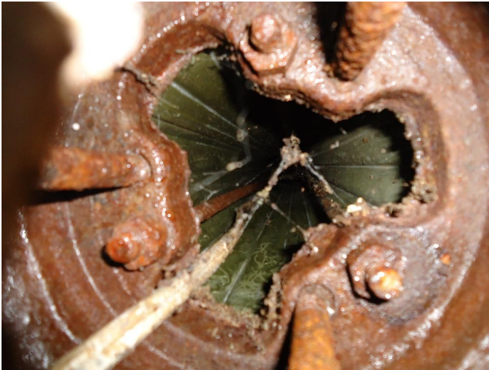
Photo 38: Moisture present in base of lamp
