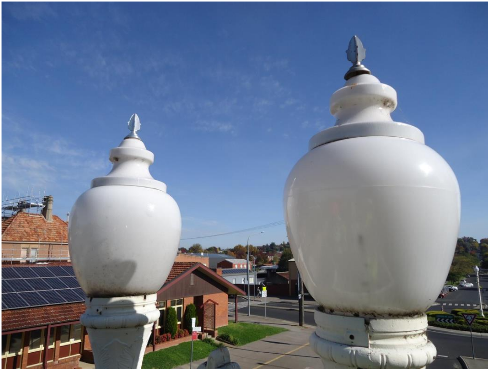
Photo 9: Skewed Finials and retaining rod resulting in poor seal and permitting water ingress and access for insects
