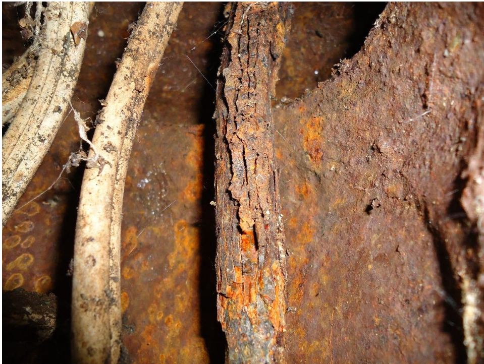
Photo 36: Corroded anchors from Machattie Park and Kings Parade Lamp Standard
