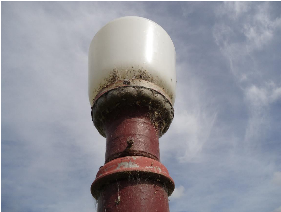
Paint flaking showing potential galvanising of cast iron Lamp Base
