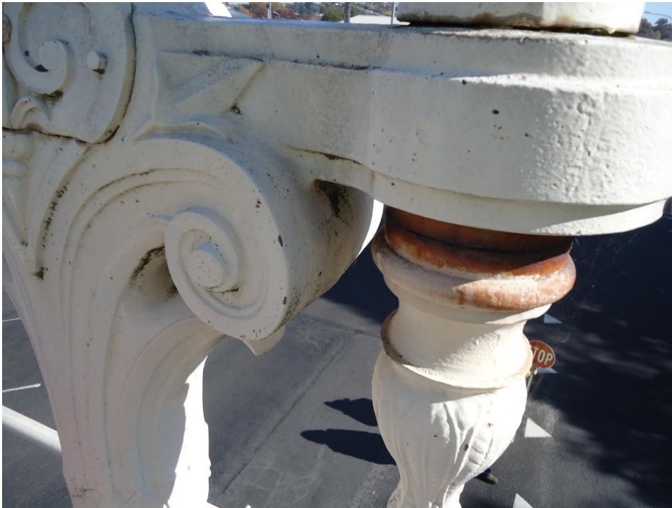
Photo 25: Corrosion at Base Finial and Centre Moulding
