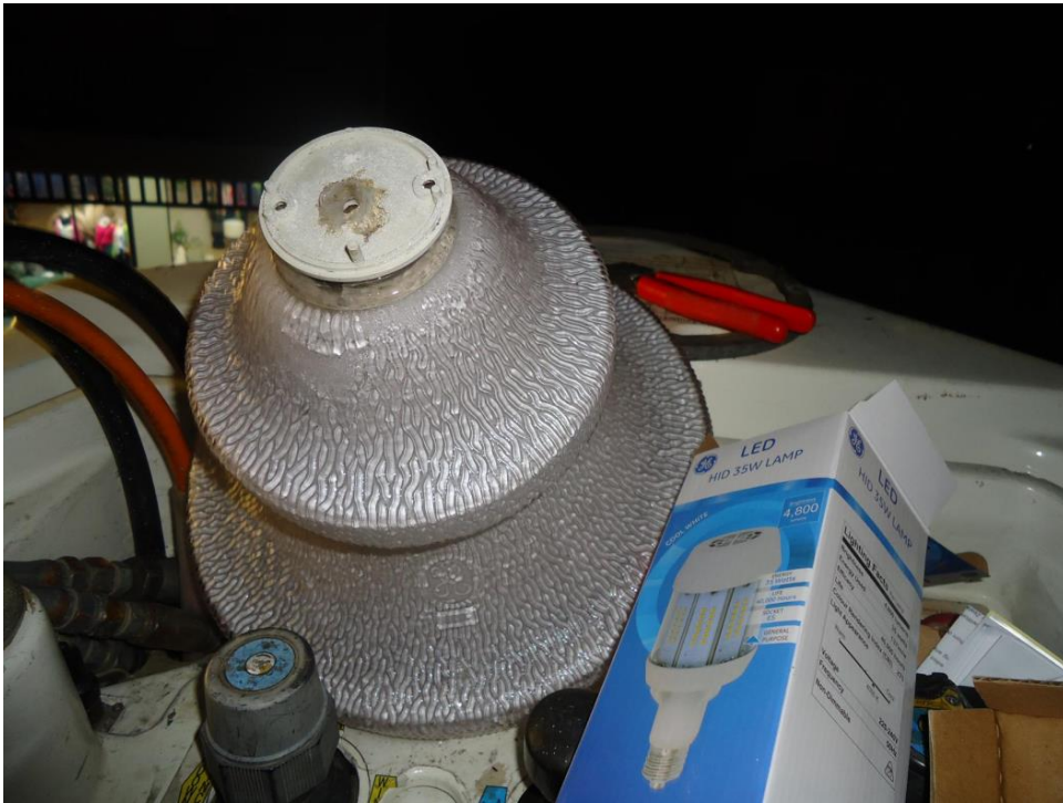
Photo 5: Attempt to seal light by previous maintenance worker where Finial was missing
