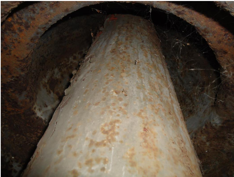
Photo 26: Surface corrosion inside of Base
