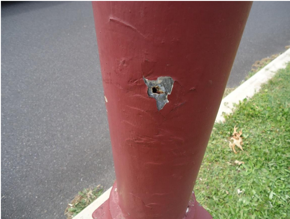
Photo 51: Thin wall galvanised post – potentially not original
