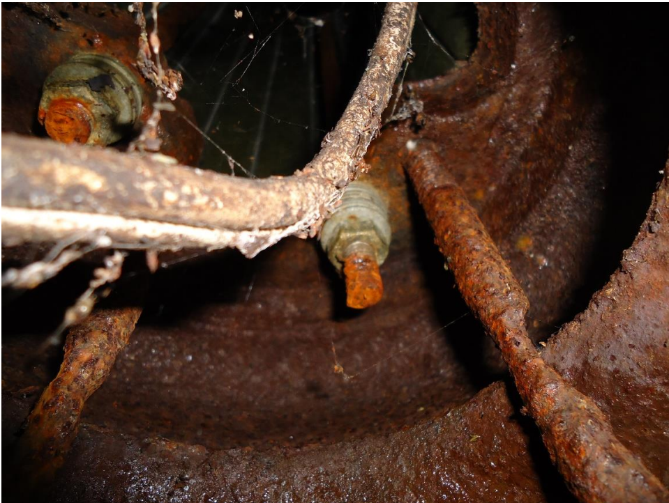
Photo 37: Corroded anchors from Machattie Park and Kings Parade Lamp Standard
