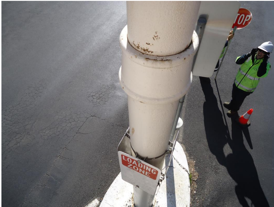
Photo 19: Mastic sealant between collar and post at the end of its life
