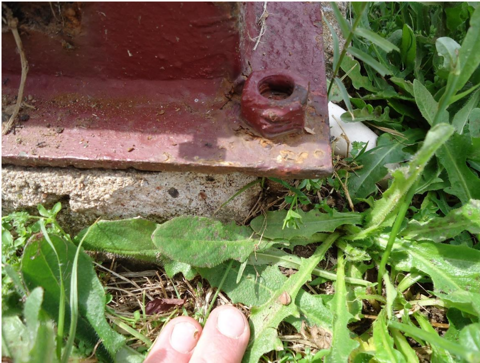
Photo 53: Ineffective fastener on same lamp as Photo 52
