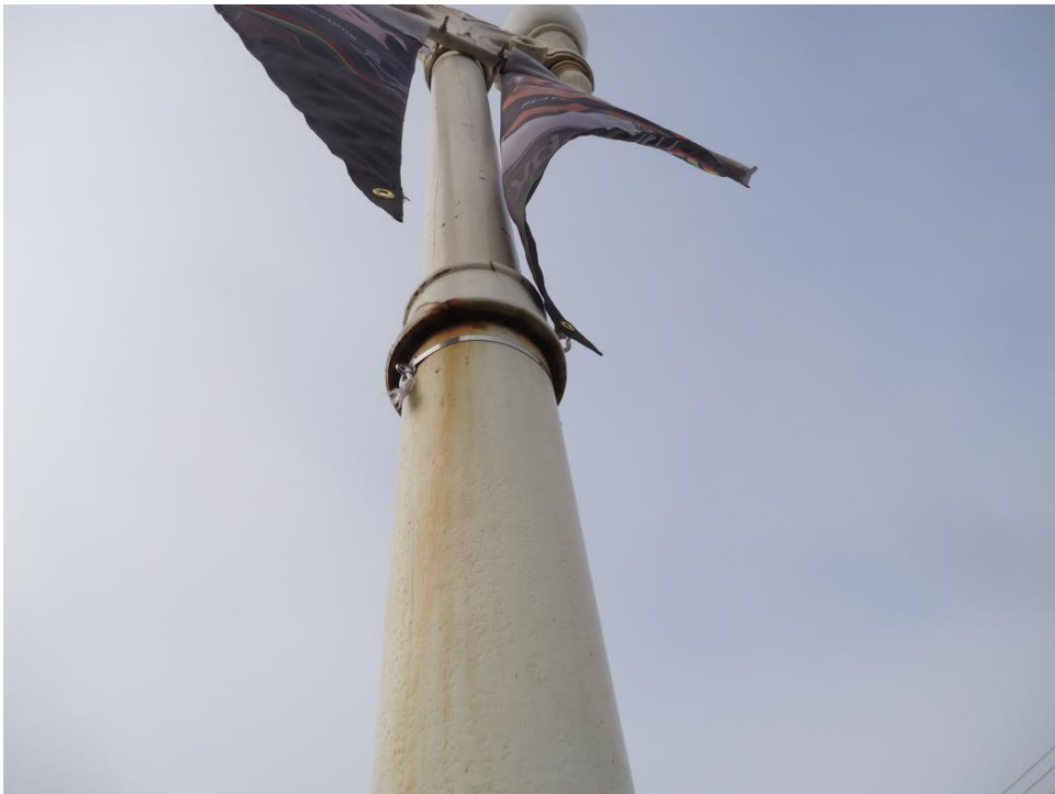
Photo 22: Corrosion from water ingress between collar
