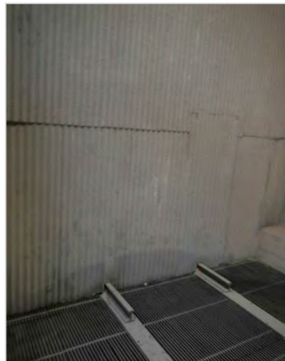
Figure 196 Railway siding—note the rails have been cut (© Kasiannan, 2015)
