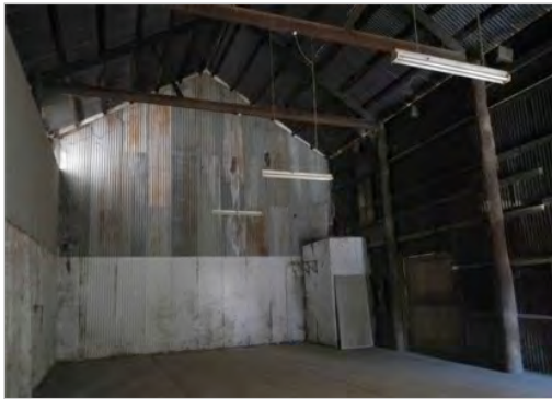
Figure 106 Shed adjacent to the railway weighbridge—note the undressed timber posts (© Kasiannan, 2015)
