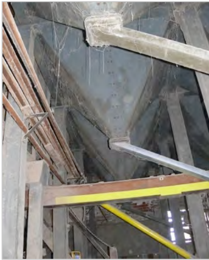
Figure 121 Lower section of the smaller 30 tonne oregon silos (© Kasiannan, 2015)
