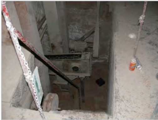
Figure 117 Tunnel linking to the space under the larger 90-tonne timber silos ;used to convey the grains (© Kasiannan, 2015)
