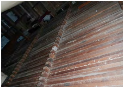
Figure 183 Mill building—second floor timber silos (© Kasiannan, 2015)
