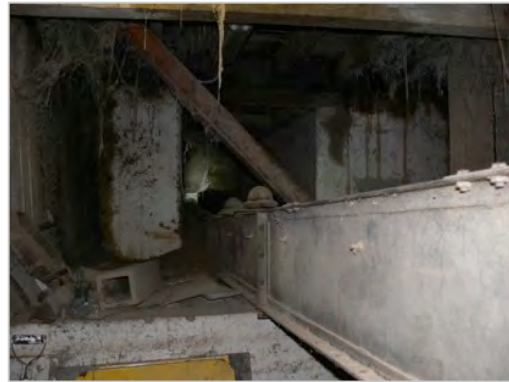
Figure 118 Tunnel linking to the space under the timber silos used to convey the grains (© Kasiannan, 2015)
