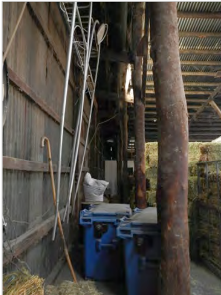
Figure 103 Bedwells Feed Barn interior—undressed tree trunk column (© Kasiannan, 2015)
