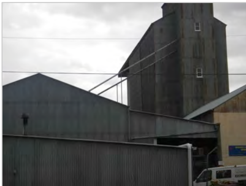
Figure 216 Large shed to the rear—note the pipes connecting to the shed roof from the silos (© Kasiannan, 2015)
