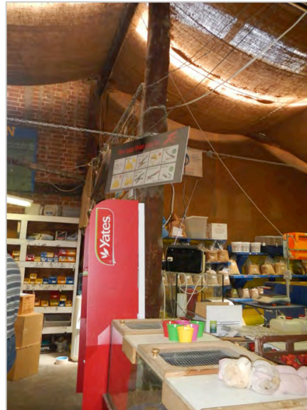
Figure 104 Bedwells Feed Barn interior—older section to the left and later addition to the right. The brick wall stops at the line of the undressed timber columns (© Kasiannan, 2016)
