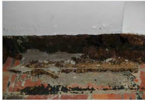
Figure 254 Cork lining used when the building was used for cold storage (© Kasiannan, 2015)
