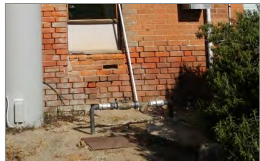
Figure 77 Loss of mortar between the bricks along northwest corner of the building (© Kasiannan, 2015)
