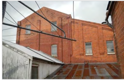
Figure 135 Mill building from the rear of the Victoria Stores building—Difference in brickwork indicates later additions (© Kasiannan, 2015)
