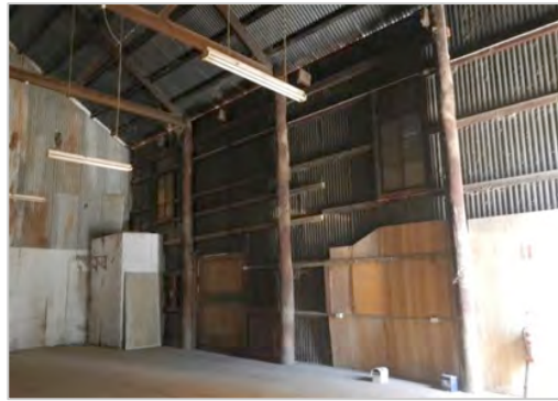
Figure 107 Shed adjacent to the railway weighbridge—note the undressed timber posts (© Kasiannan, 2015)
