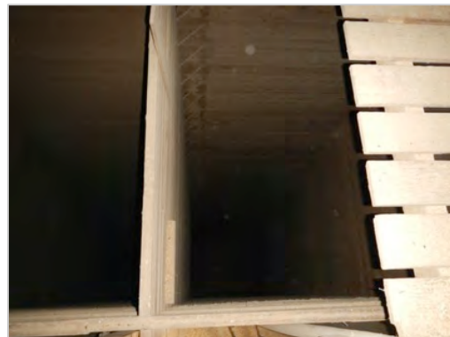
Figure 230 Interior view of timber silos—note the rungs in the corner for access (© Kasiannan, 2015)
