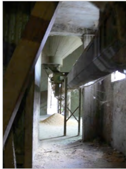
Figure 243 Pipes to carry the grain from the concrete silos (© Kasiannan)
