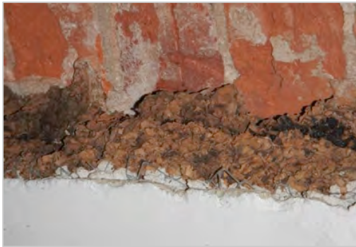
Figure 253 Cork lining used when the building was used for cold storage (© Kasiannan, 2015)
