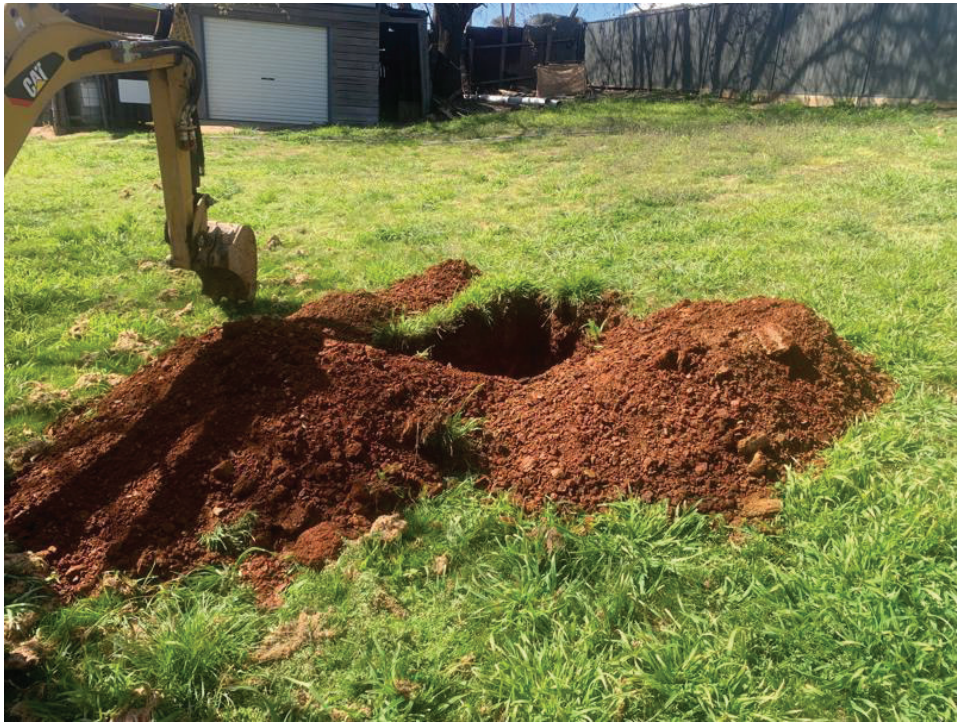
Image 1: Subsoil investigation at the proposed development site
