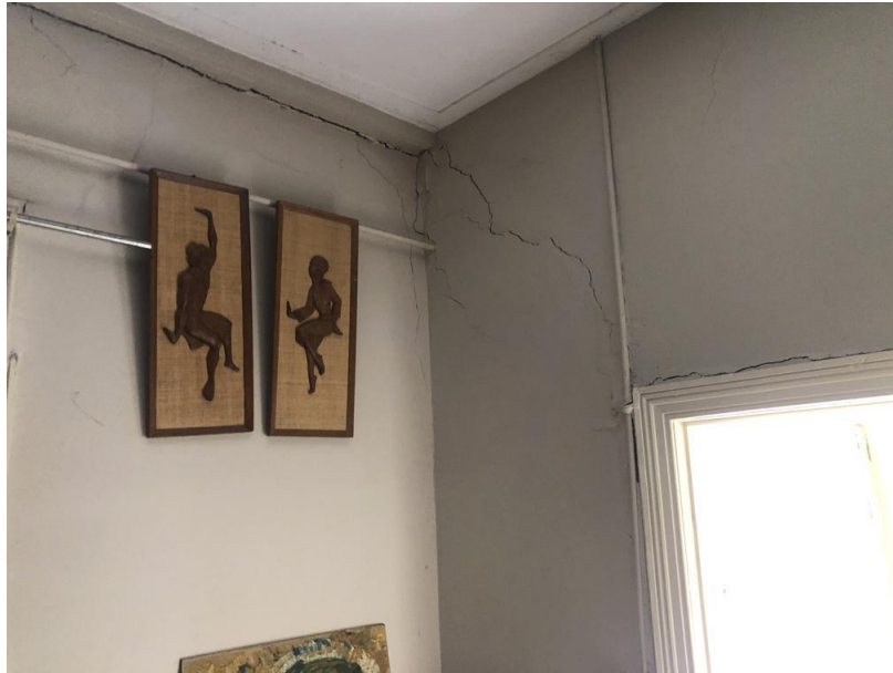
Internal wall cracking example
