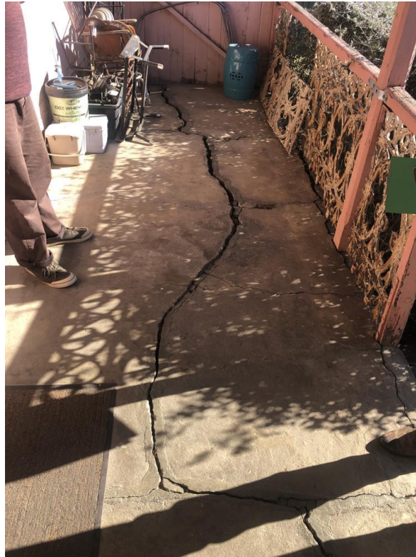
Cracking along verandah slab
