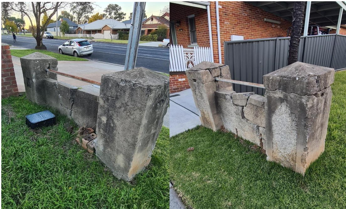
Front Fence damage example
