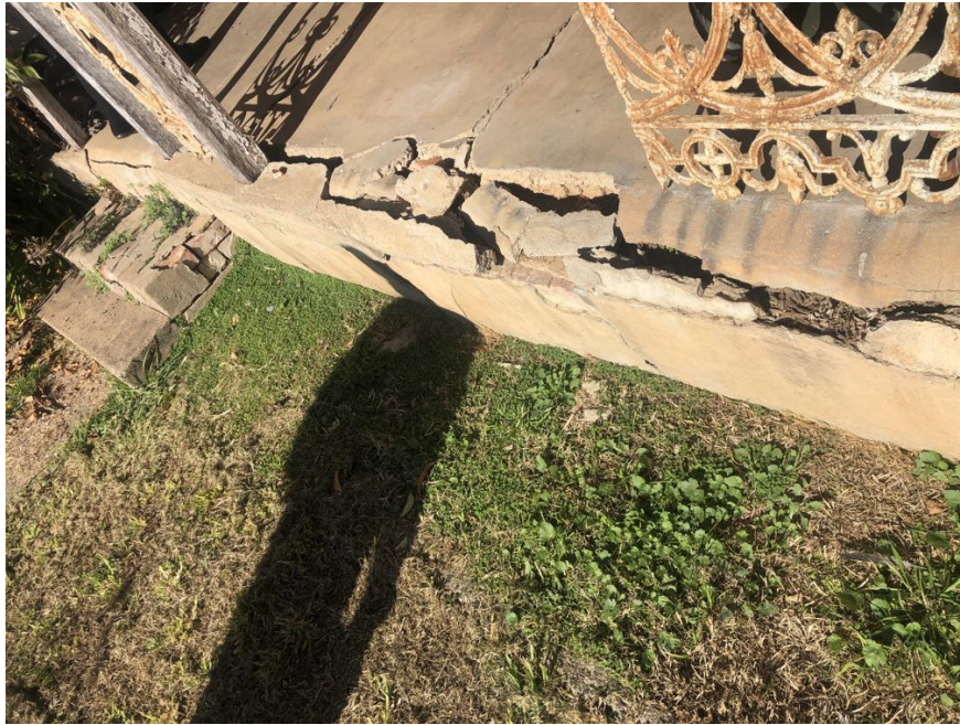
Damage to verandah slab edge
