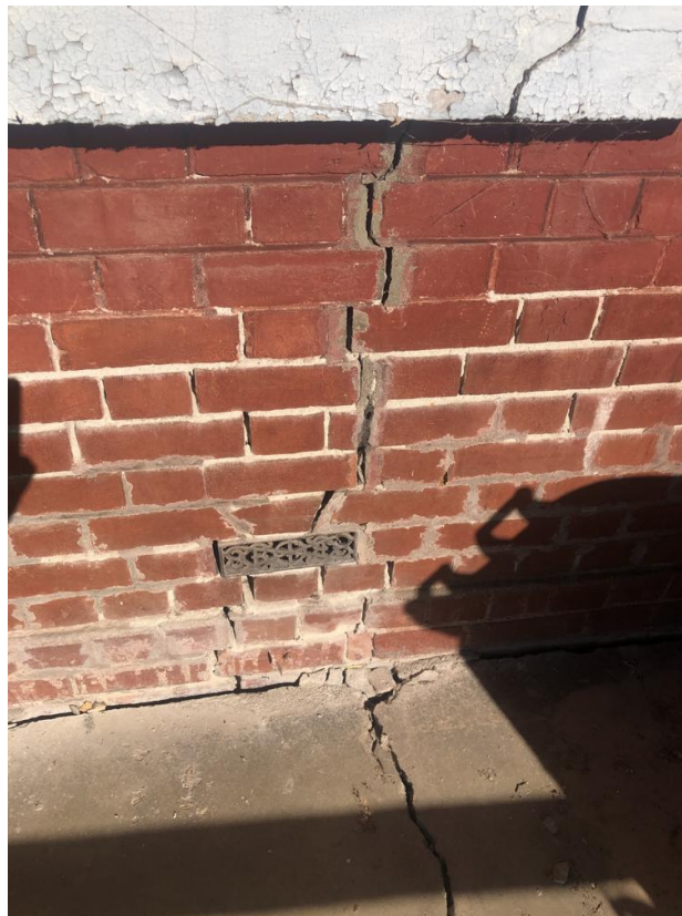
External wall cracking
