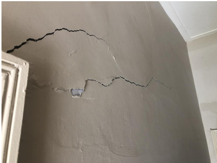
Internal wall cracking example
