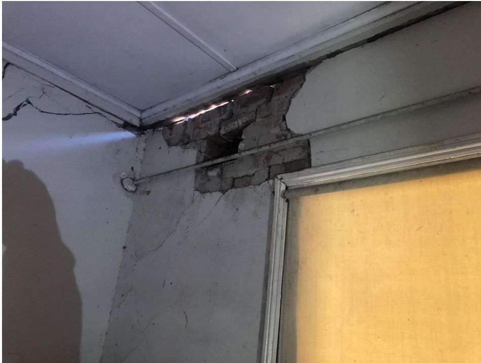
Internal wall cracking example
