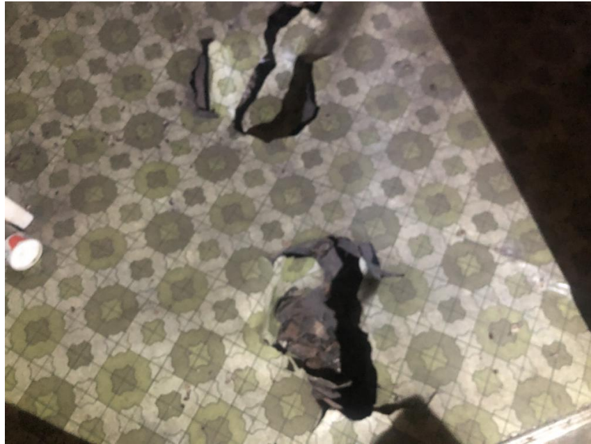
Internal floor damage example
