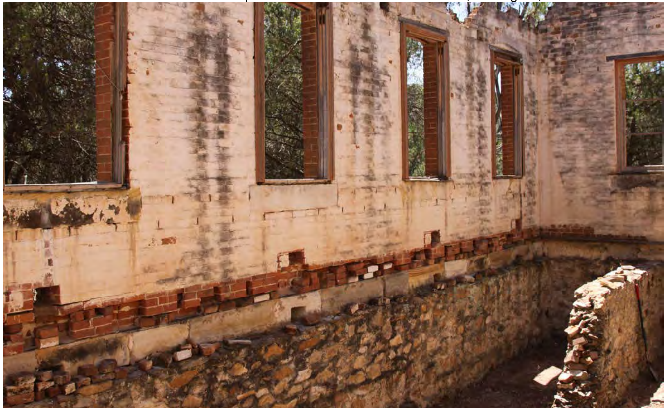
Internal view looking north (west); unpainted bricks indicate the relative level of the missing timber ground floor
