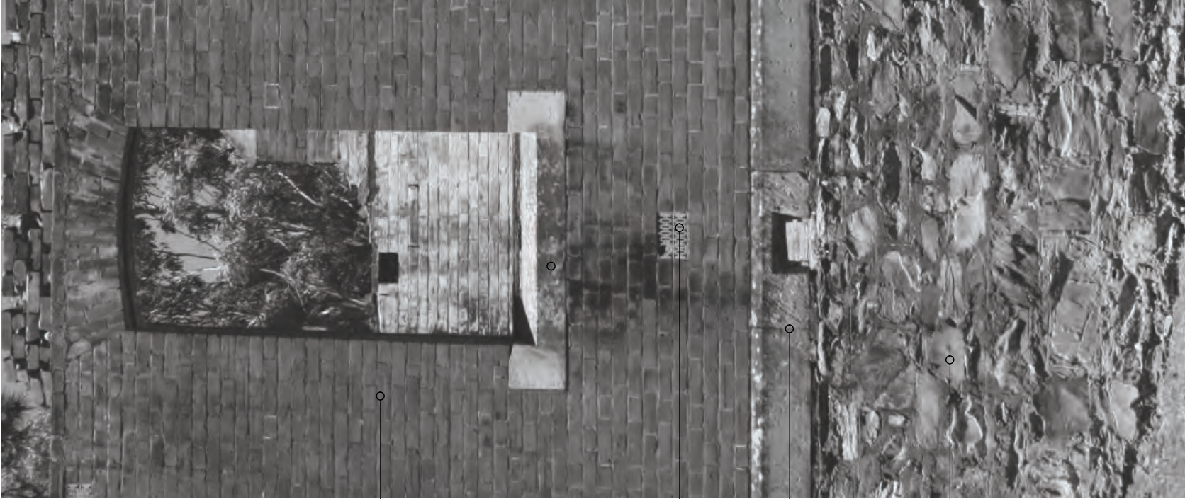
EXISTING BRICK WALLS TO BE CLEANED AND MORTAR TO BE REPLACED IF NECESSARY
