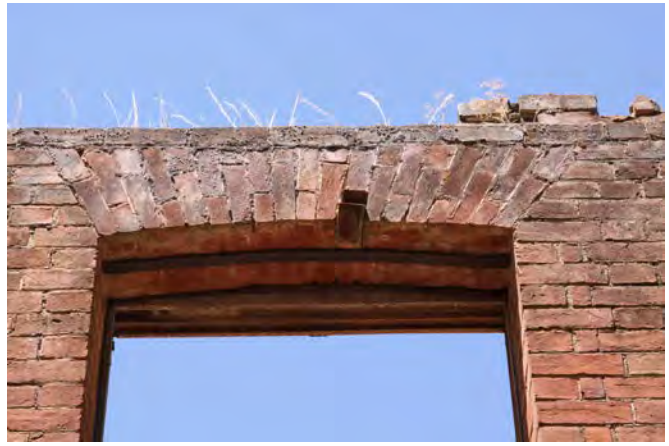
Arch detail above long façade window
