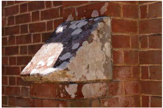
Detail of sandstone capping piece
