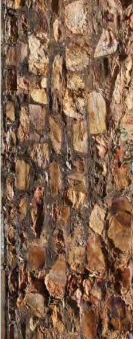
STONE WALLS NEW RANDOM RUBBLE FOUNDATION STONE WALLS TO MATCH EXISTING [S]
