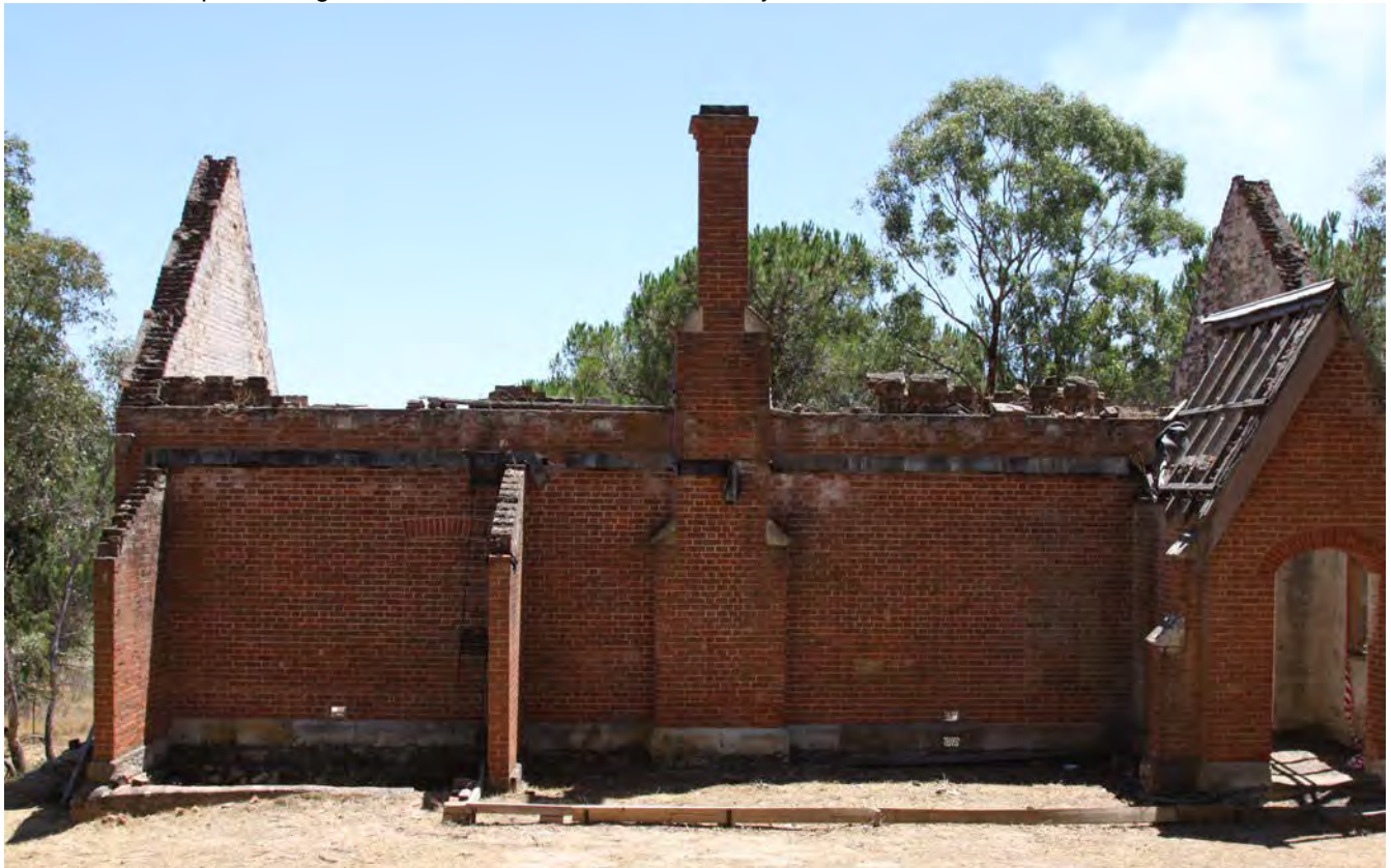
East Façade showing Entry vestibule, fire place chimney & position of former external lean to roof
