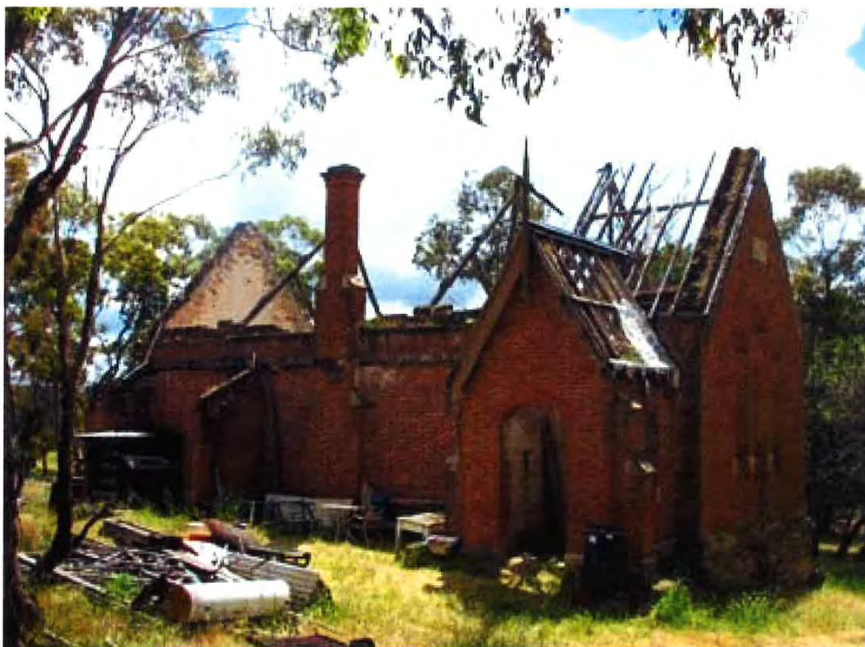
Figure 4 – Cow Flat School building with collapsed roof (after 1985)
