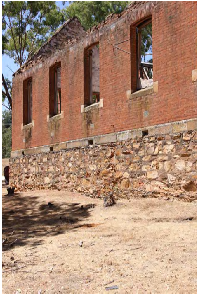
West façade with high side of random rubble plinth
