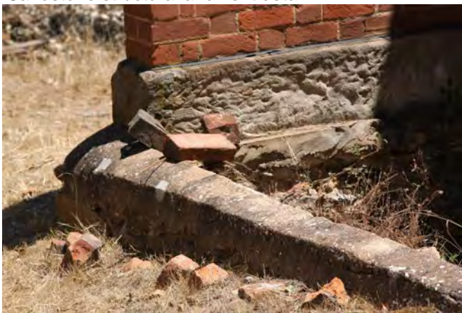
Sandstone coping detail
