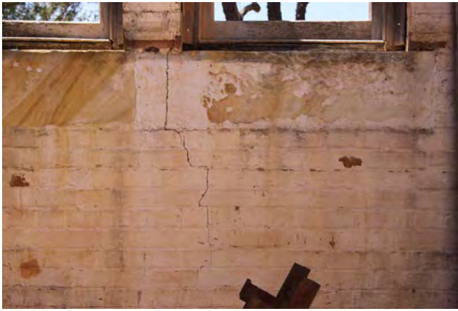
Example of minimal brick work cracking
