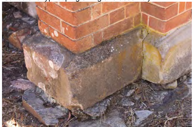
Sandstone coping / foundation detail
