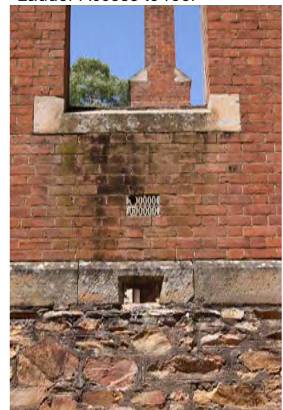
Sandstone sill and vent openings
