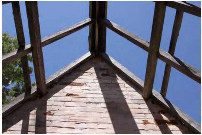
Entry vestibule roof timber structure
