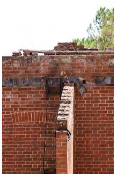
Opening bricked shut
