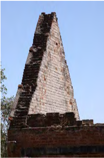
4 Brick thick gable end walls
