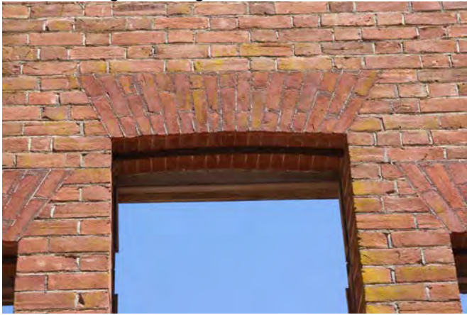
Arch detail above central gable end wall window
