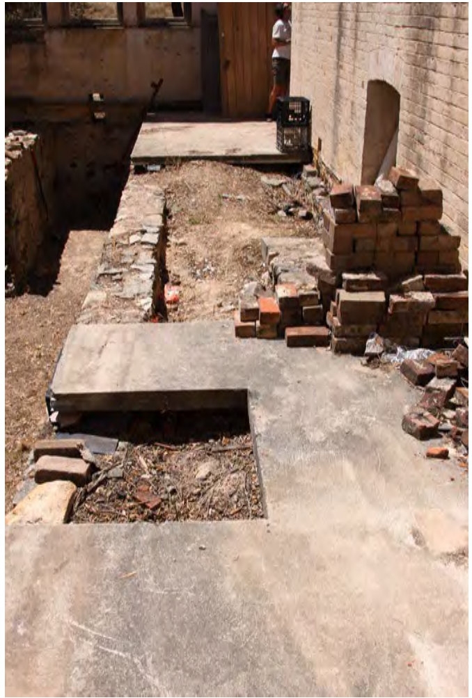
Partial concrete slabs, not original, to be removed
