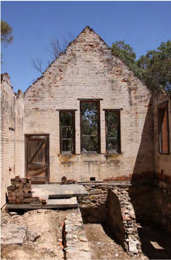
Internal view with rubble wall in subfloor space
