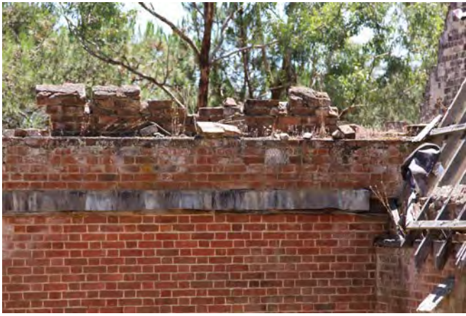
Lead flashing indicating connection of lean-to roof
