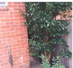
Some vegetation was found to be very close to building foundations, which could affect structural performance and damage plumbing.
