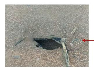
The unsealed road surface of William Lawson Drive has eroded and 'caved in' allowing sedimentation to flow into the culvert drainage system
