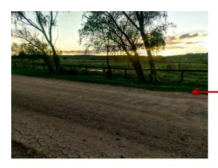
Sedimentation from the unsealed William Lawson Drive runs off as a result of the natural drainage in the area into our dam and then into the river
