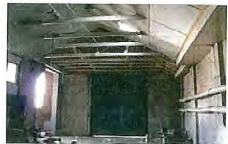
Figure 3.19- Building 4 interior, looking south, showing timber trusses, ceiling and roller shuttered opening on front facade
