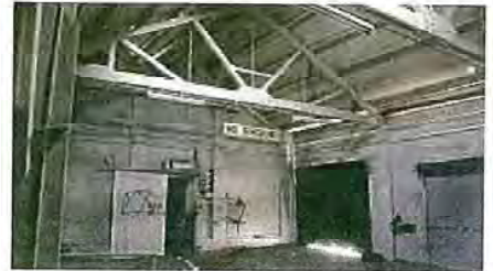
Figure 3.14- Building 2 interior showing 'Howe' timber trusses with steel rods common to other buildings on site
