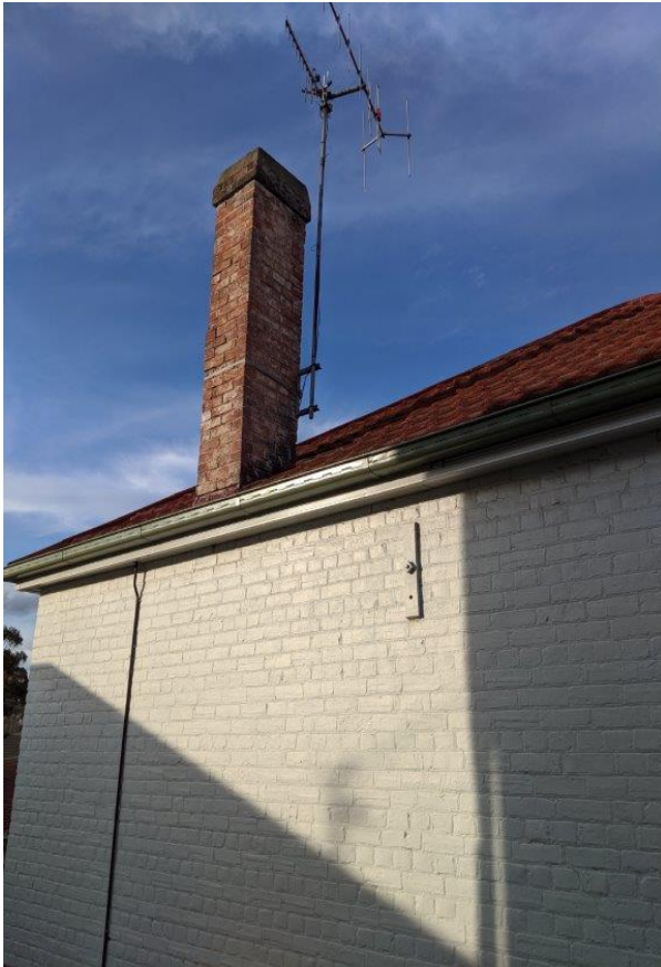
Image 15 A detail view of the brick bonding consisting of three stretcher courses and one header course which is known as Flemish garden wall bonding. Note the damaged brickwork in the chimney flue. Restoration of the brickwork and re-pointing will conserve the two chimneys.
