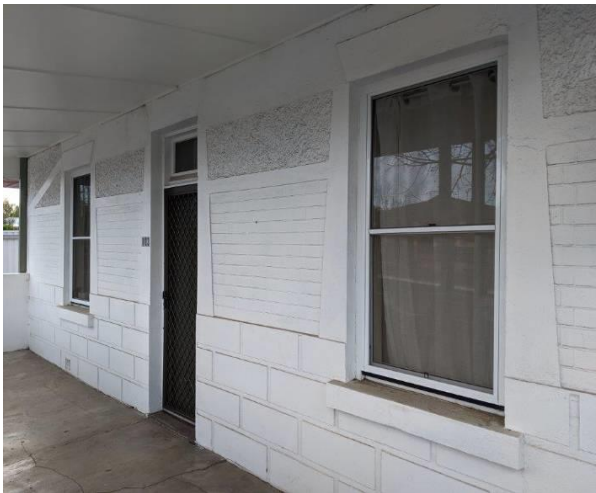
Image 13 The ashlar cement rendered dado wall treatment, inter-war inclined window surrounds to the aluminium double hung sliding sash and roughcast panels to the front facade.
