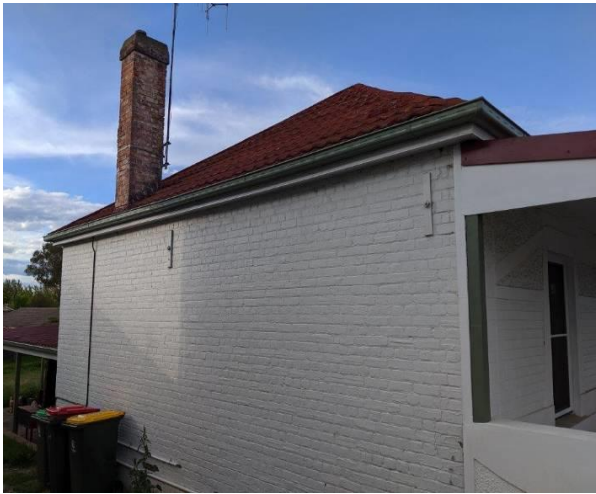
Image 16 A general view of the West Elevation, noting the wall tie rods, damaged chimney brickwork and the metal roof – ‘Decramastic’ tile sheeting provided to emulate a tile roof.
