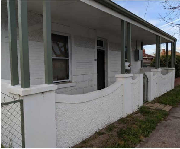
Image 12 A detail view of the cottage verandah with roughcast rendered waist high wall to the verandah
