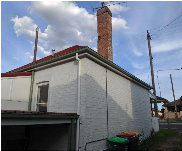
Image 18 General view of the rear North west corner of the cottage noting the simple four room bulk which sits beneath the hipped roof with the timber framed rear skillion to the rear.
