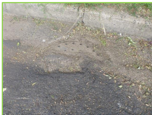
Buried sewer manhole, Beside 212 Rankin Street
