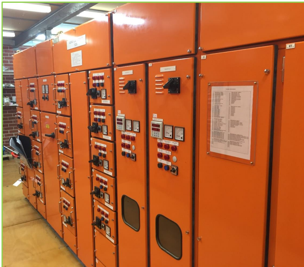
Switchboards in Control Tower, Wastewater Treatment Plant
