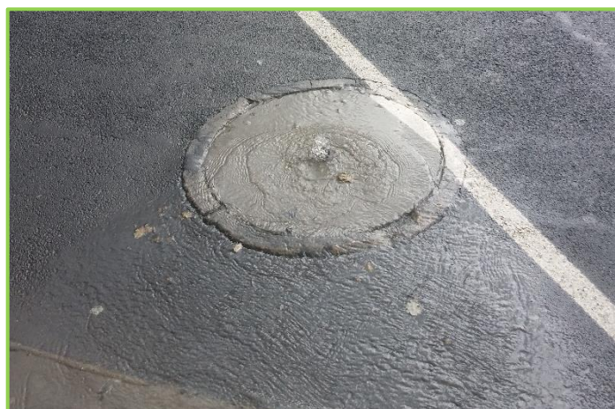
Surcharging sewer manhole, George Street
