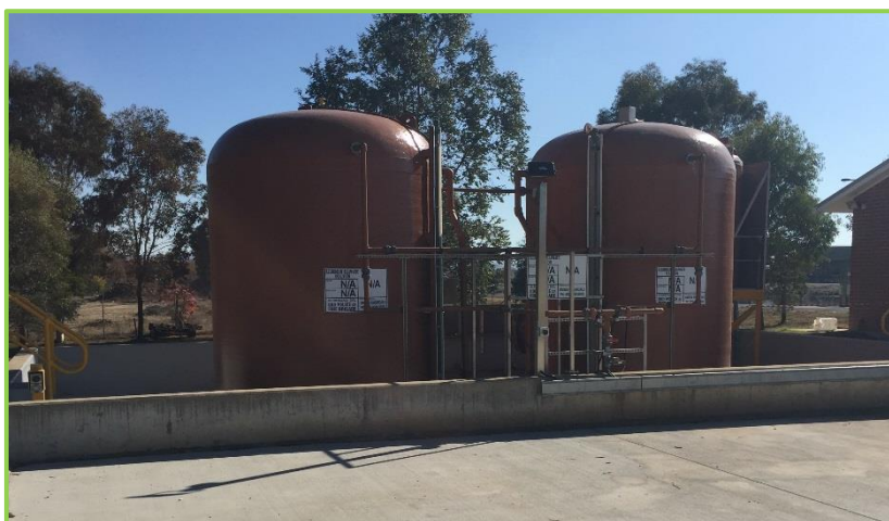
Aluminium Dosing Plant, Wastewater Treatment Plant
